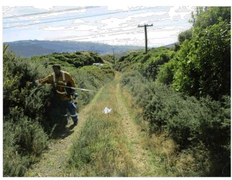
Plate3: Measuring tape showing a four metre width of a section of the access track that would be used to install the 11kV cable underground . 29 March 2019.
