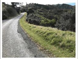
Photograph 3-10: Typical alignment showing patching to edge break
