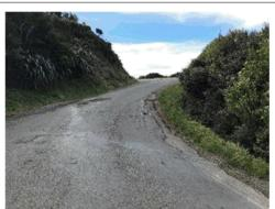
Photograph 3-6: Cracking and edge break
