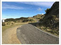
Photograph 3-14: RoW south towards Radome, metalled widening on corner with repaired edge break
