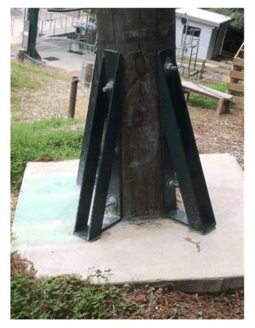
**Figure 14:** Alternate pole footing option. This requires less excavation and soil removal and simply requires a 500mm thick concrete pad to be laid. Note: This is an option for this project but not until proper design projects have been completed would this type of detail be confirmed.
