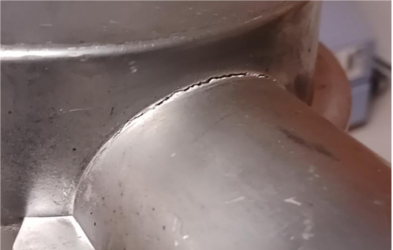
Figure 16 – New spigot failure
