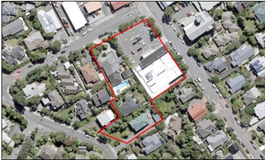
Figure 1: Aerial view of the subject site and the surrounding environment.
