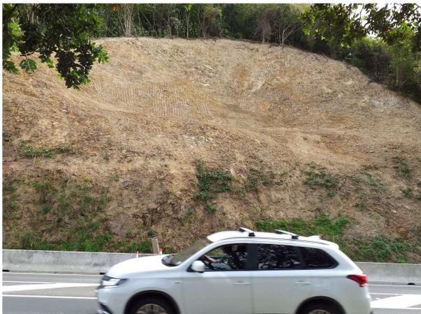
3. **Earthworks** do not comply with the district plan. **The proposed 697m<sup>2</sup> exceeds the permitted 250m<sup>2</sup> by 178.8%**. The excavation depth also (1.6m) exceeds the permitted 1.5m. This could also have an adverse effect on the stability of the site.
