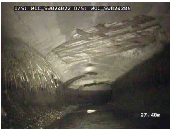
WCC_SWP025801_b67022bc-c7a1-4f64-981d-72f80bee0da8_20211203_115723_284.jpg, 00:07:27, 27.40m Obstruction permanent, reduction of up to 10% of the pipe diameter from 11 o'clock to 1 o'clock / REINFORCED CONCRET SLAB?
