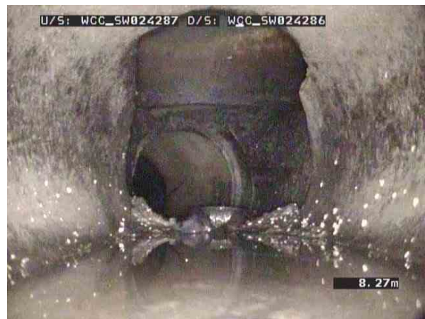
WCC_SWP025804_6295fca4-a9ba-413b-936a-9f7bf3569196_20211203_134529_352.jpg, 00:04:43, 8.27m General comment / EELS IN PIPELINE
