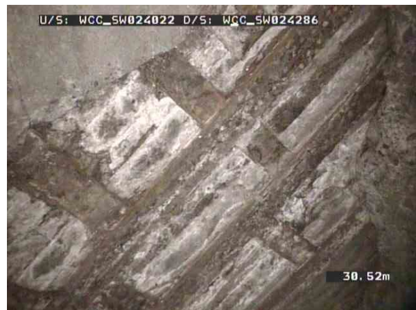
WCC_SWP025801_4da97f73-fc7c-437a-8d5f-8b43f2c9b4ac_20211203_115802_728.jpg, 00:07:27, 27.40m Obstruction permanent, reduction of up to 10% of the pipe diameter from 11 o'clock to 1 o'clock / REINFORCED CONCRET SLAB?
