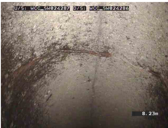
WCC_SWP025804_14e520b2-e007-4add-bc6b-7ee710cc7776_20211203_134315_289.jpg, 00:04:15, 7.66m Crack circumferential, crack, large, open and there is evidence that it extends through to the outside wall from 9 o'clock to 3 o'clock / ED FROM CRACK
