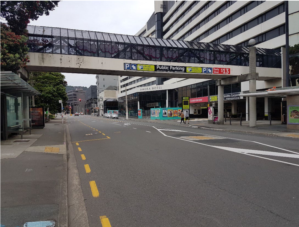
Figure 4: View east along Wakefield Street (Development Site on the left)
