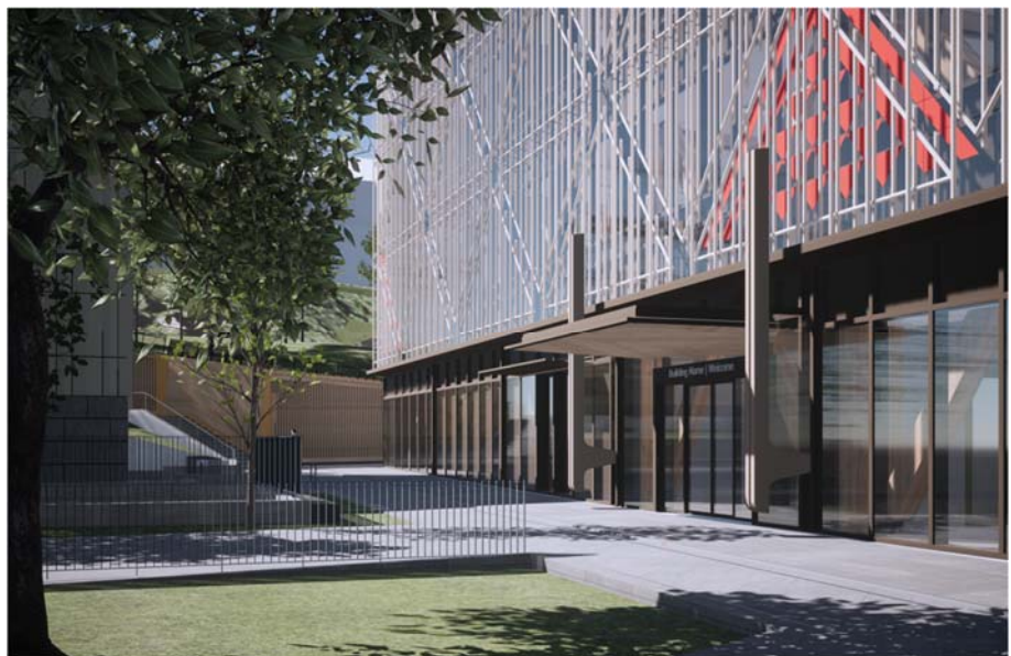
Figure 3. View of MUS enlarged west entry canopy with glass wind screens. Note that the red frit on the glass visible above the canopy will in fact be white.
