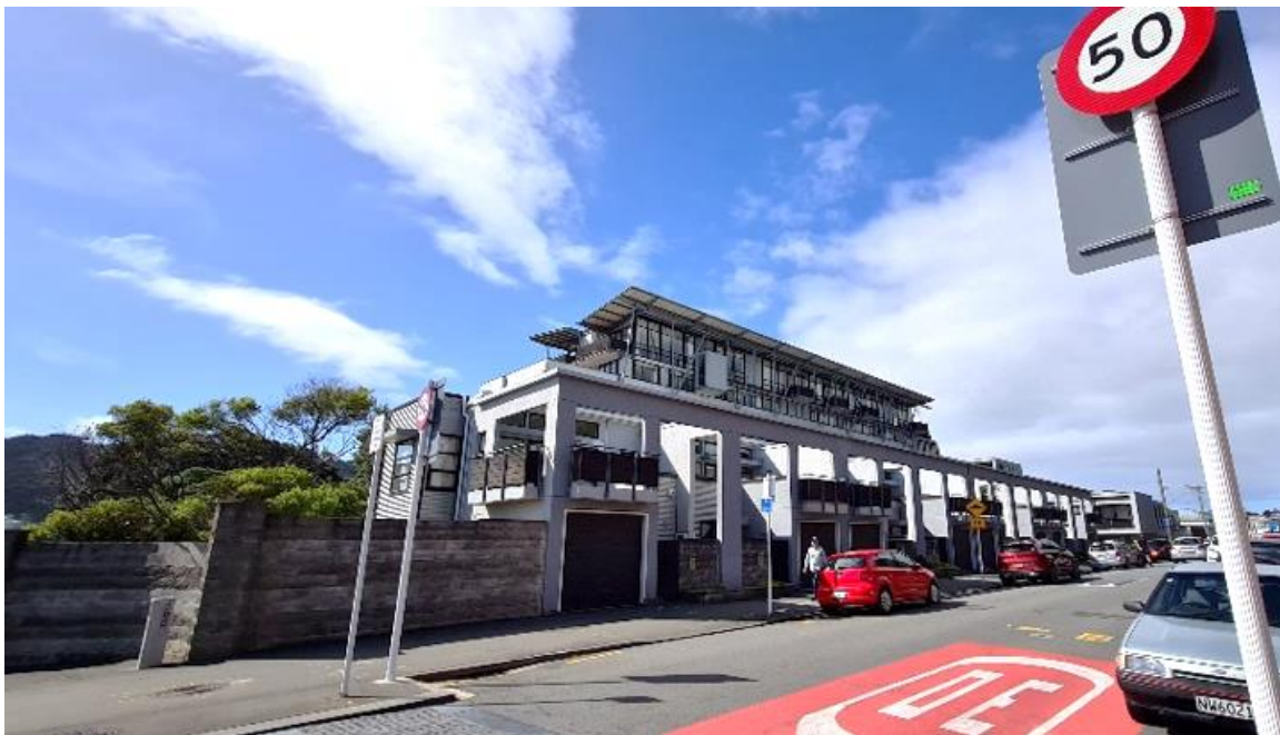
Figure 6: Existing townhouses along Tasman Street
