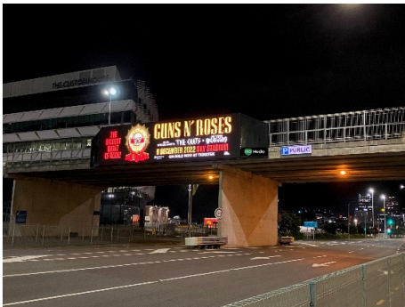
3. Waterloo Quay Overbridge (North)
