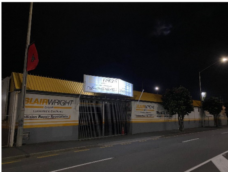
5. 89 Waterloo Quay (Internal Lighting)
