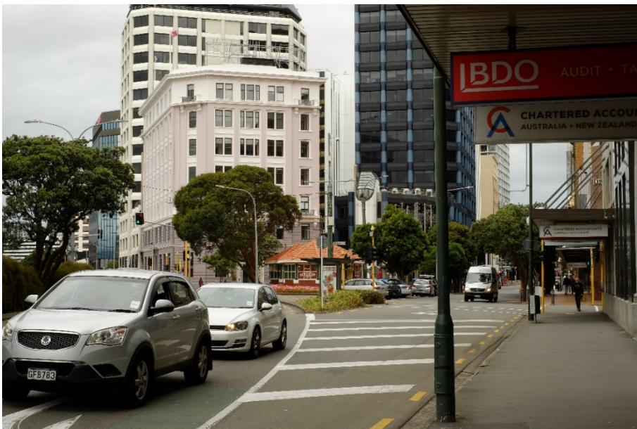
Figure 4: View of the building from the north (from west side of Customhouse Quay) (photo RKL 7th February 2022)
