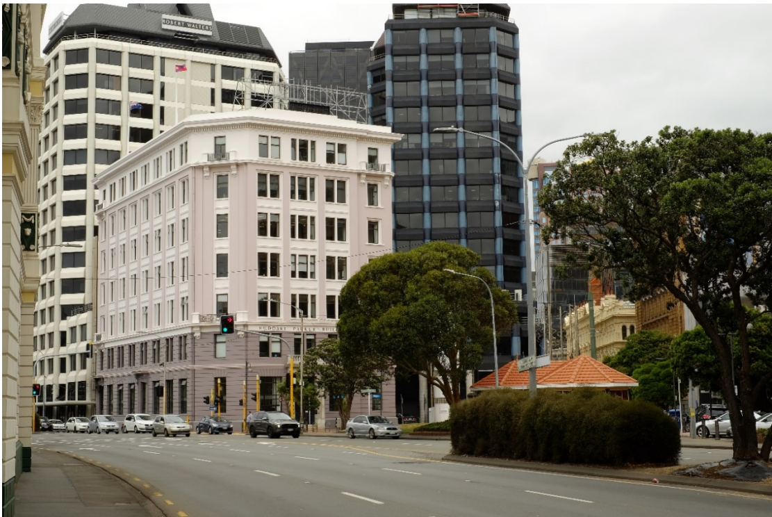
Figure 2: Building as existing with structure to support sign at roof level (photo RKL 7th February 2022)
