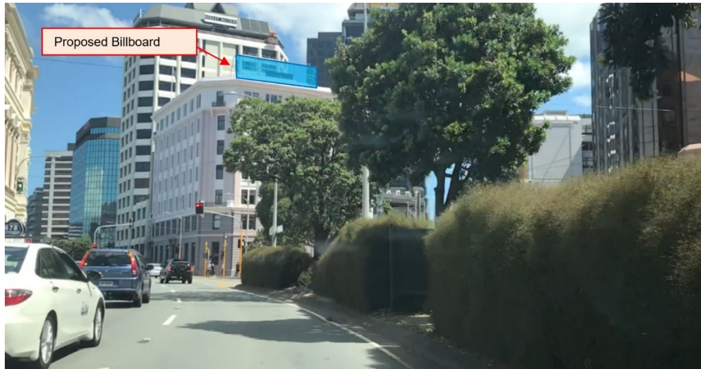
Figure 3: Southbound view at ~80m
