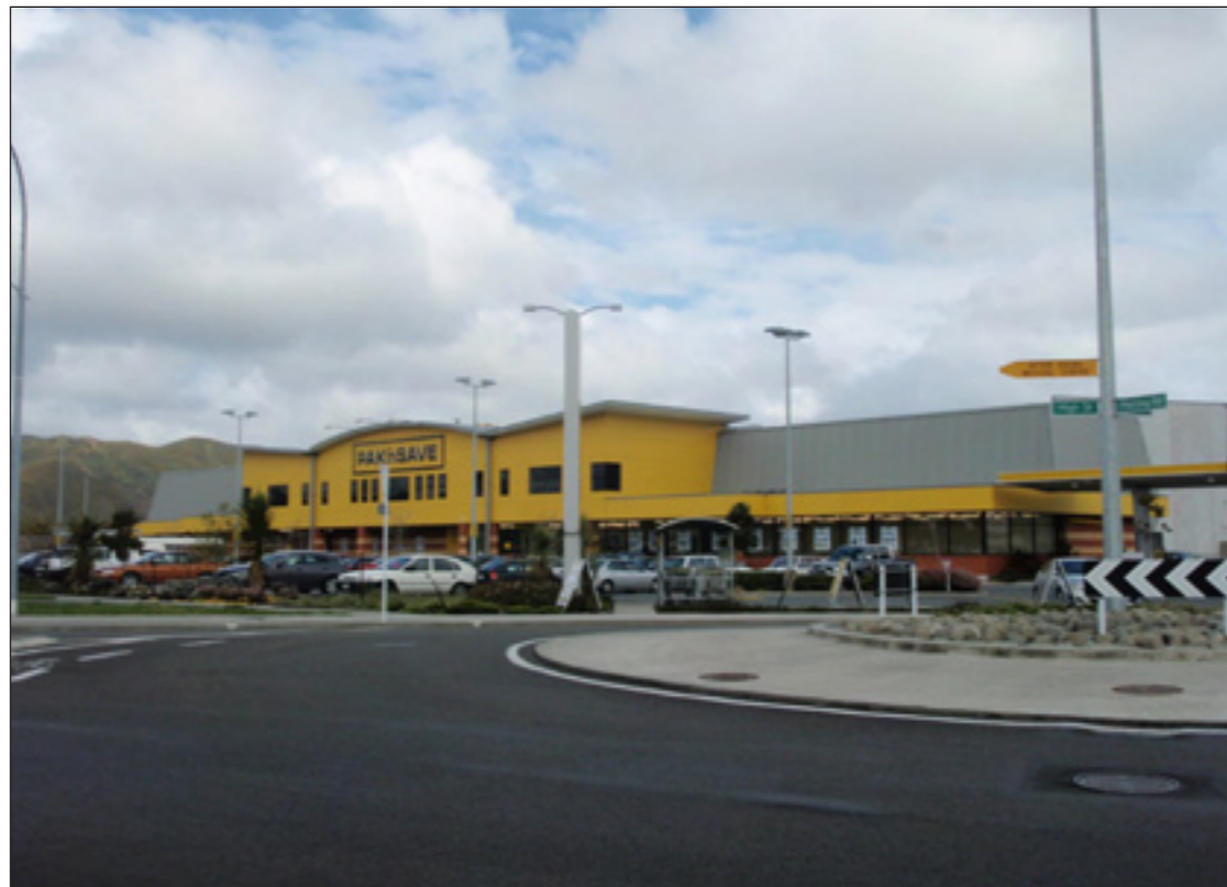
Typical scale of commercial and industrial activity and structures in the area
