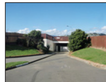
The pedestrian underpass connecting Coutts Street to Miramar.
