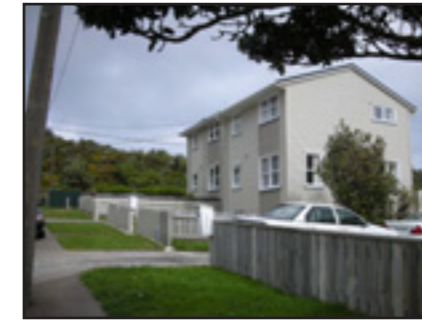
Some of the houses in Kekeranga Street have an identifiable state house style.
