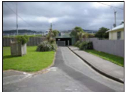
The pedestrian underpass connecting Coutts Street, Rongotai to Miro Street, Miramar.
