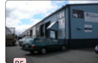
B5 INDUSTRIAL BUILDING
