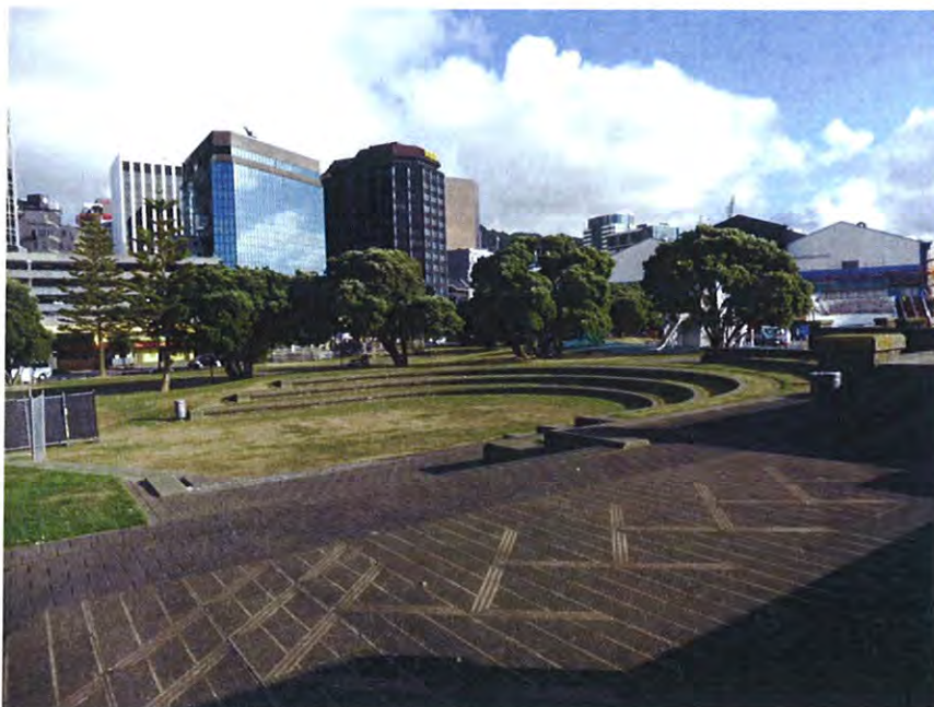
PHOTO 2: existing 'amphitheatre' and steps and harbour facing wall which are to be removed and 'replaced' by the Harbour Lawn
