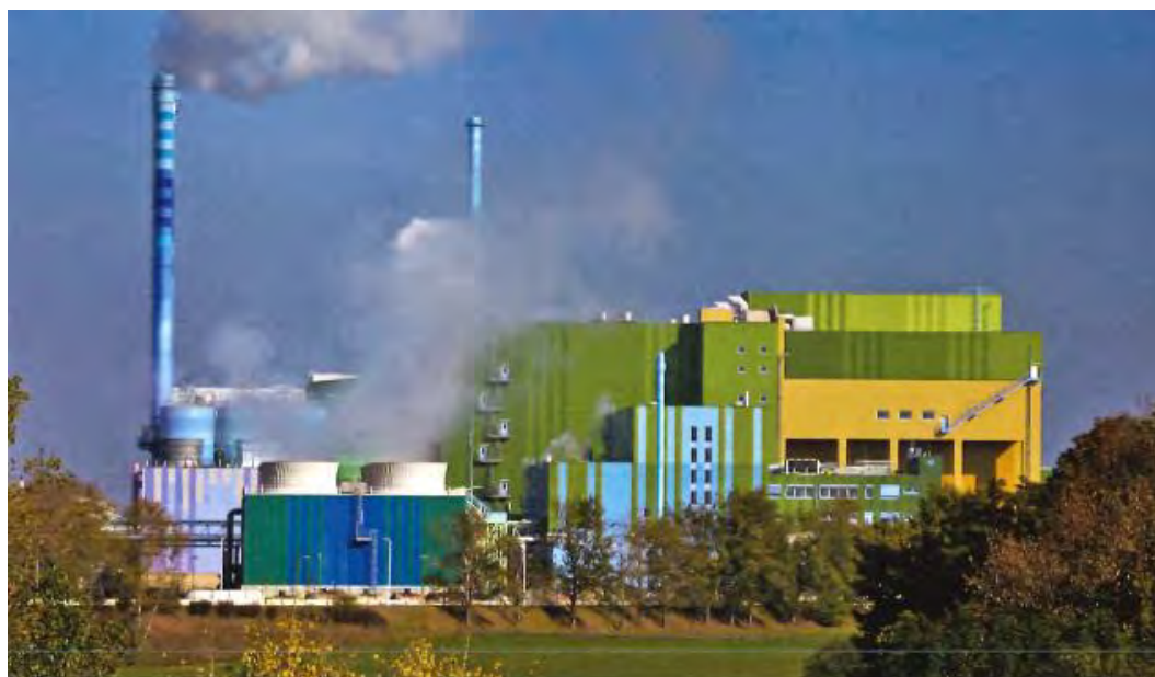
Figure A1.1 Energy from waste facility 18
