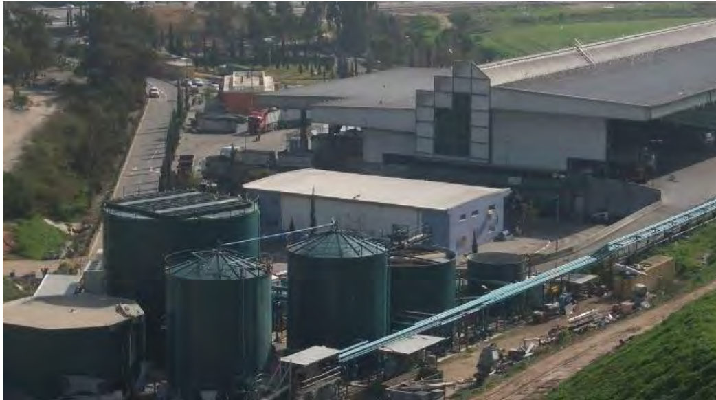
Figure A4.1 Mechanical Biological Heat treatment facility 27
