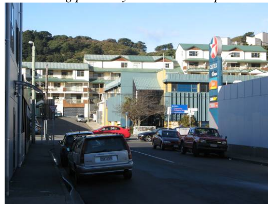
Mix of building types, viewed from King Street
