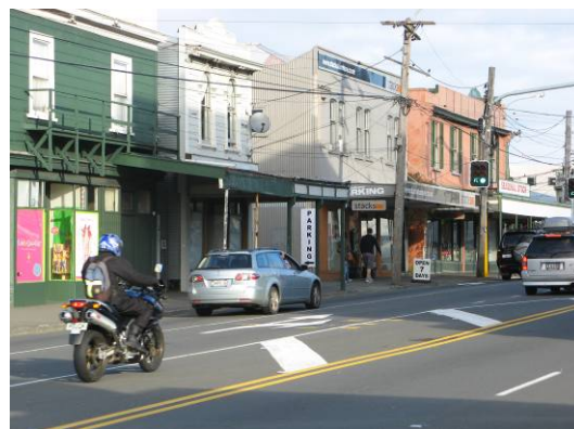
Modest, narrow-fronted old buildings form a traditional streetscape close to John Street
