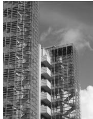
Sophisticated detailing in a contemporary building
