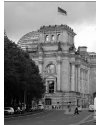
Publicly significant building demands contrast
