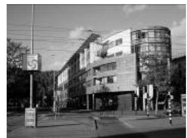
Examples of buildings defining public space, and articulation of form and façade to give visual interest
