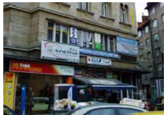
Numerous signs of contrasting size, style, type, colour and graphics, viewed in close proximity, add to the collective effect of clutter
