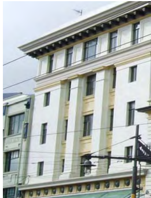
Architectural features (defined in section 4) help to 'sub-divide'/articulate the building façade and provide visual interest and a sense of relief. The size, proportions and arrangement of these elements determine the architectural composition of the building façade. The intensity and imagery of the façade elements/features determine the architectural style of the building and its detailed design quality.
