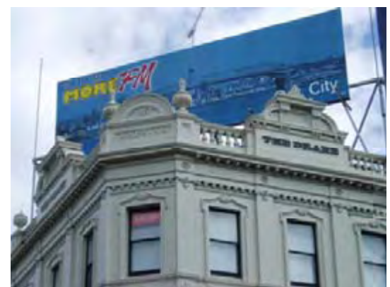
The sale and location of signs on heritage buildings should be sensitively approached. Signs projecting above the parapet line, as this one, have a significant impact on the heritage value of the building, altering its silhouette line and compromising its overall quality
