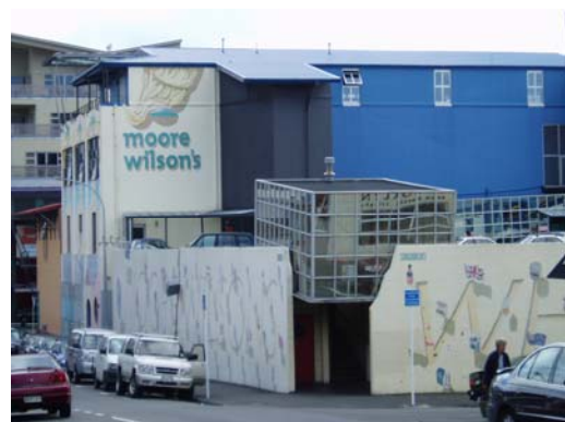
Visually interesting, innovative signage can enhance the building image and add vitality to the streetscape
