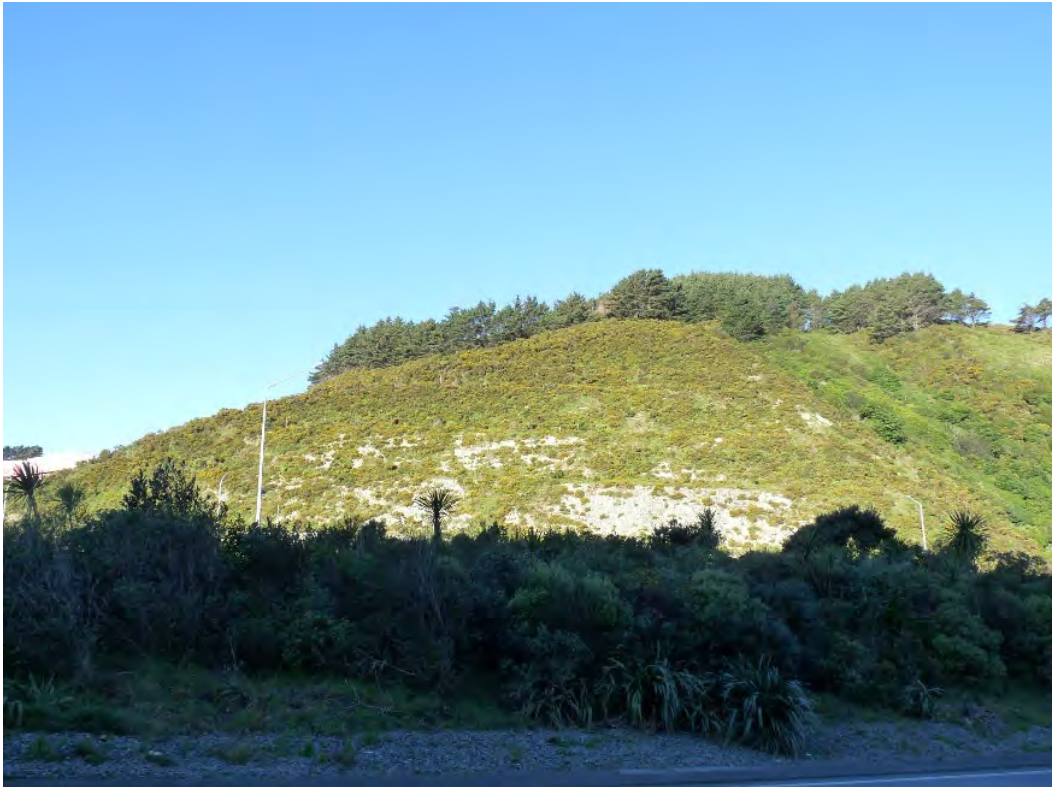
Photo 3: View towards road batters at Newlands Interchange, July 2018
