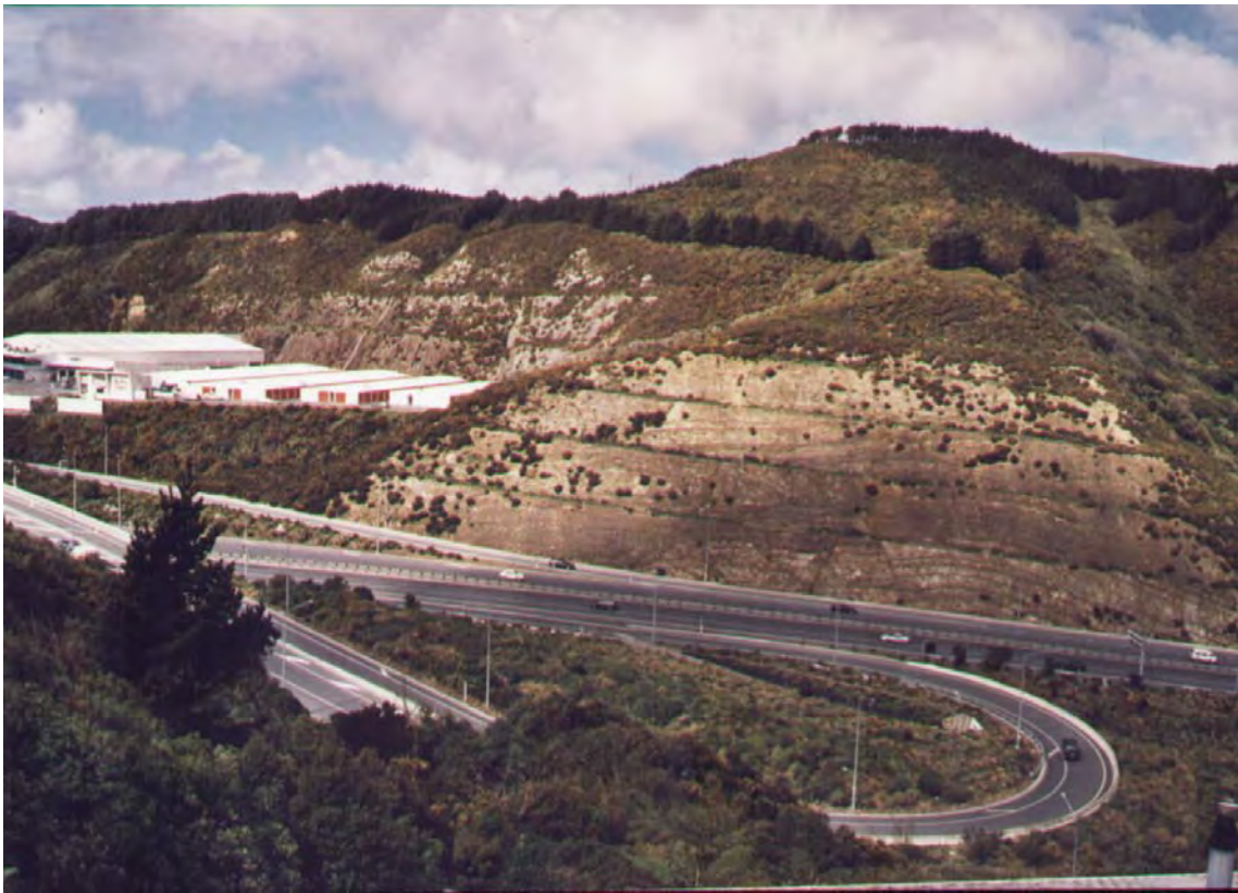
Photograph 5 : Newlands Interchange on SH1, 2003, showing recent road batters (centre) and older cut faces behind industry (centre left).
