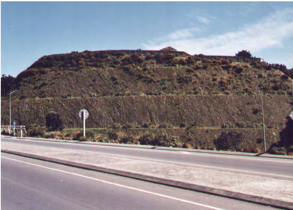
Photograph 8 : Benched road batters at Newlands Interchange. The vertical faces have been hydroseeded but plant establishment has not been aided by vertical surface scrapping.
