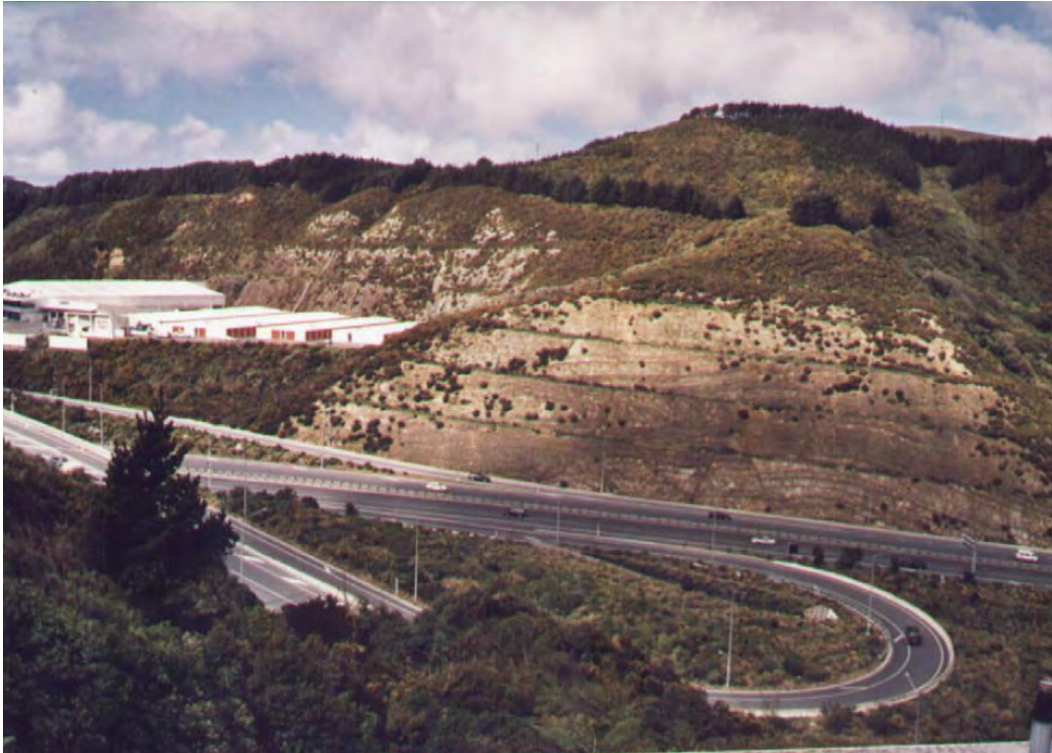
Photo 2: View towards recent road batters at Newlands Interchange, 2003
