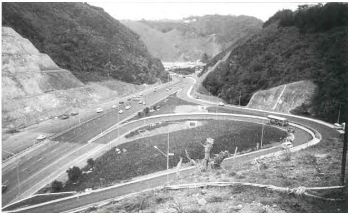
Photo 1: Newlands Interchange with road batters visible in left of view at completion, 1998
