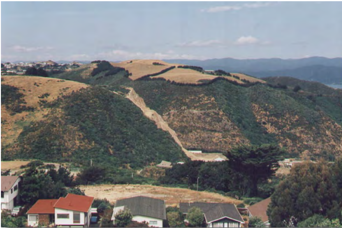
Photograph 7 : View into Ngauranga Gorge from lower Braodmeadows. Large cut faces formed during SH1 widening in the 1930-1960s are visible (centre and center right). The existing Kiwi Point Quarry can be seen in profile as a strip of recently exposed rock (left centre).
