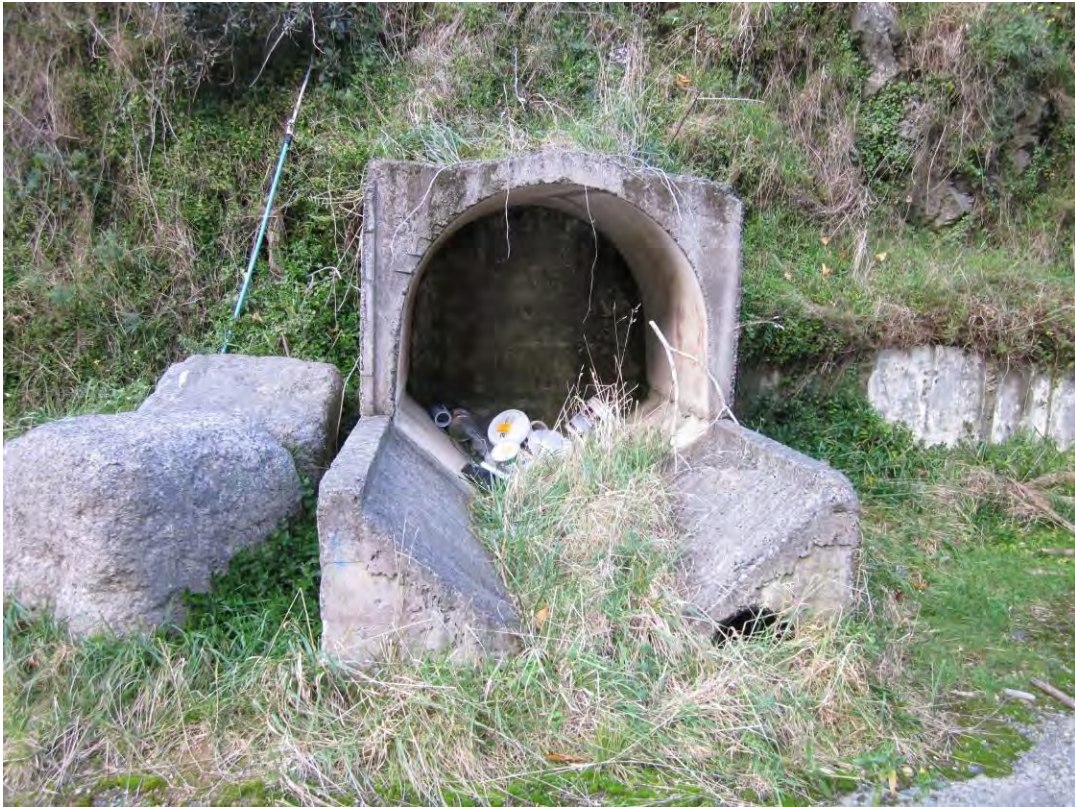
Photograph 6 Example obstructions to be expected in the fills
