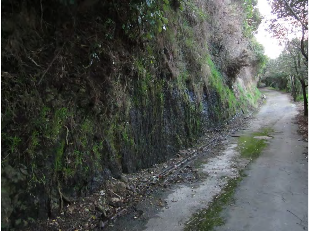
Photograph 4 Steep rock cut adjacent to Old Karori Road
