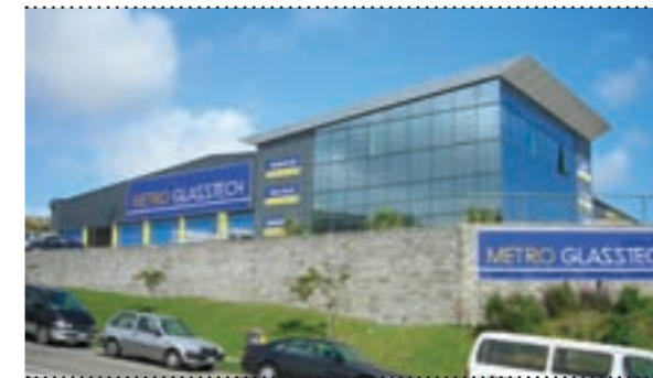
INDUSTRIAL BUILDINGS, GRENADA NORTH
