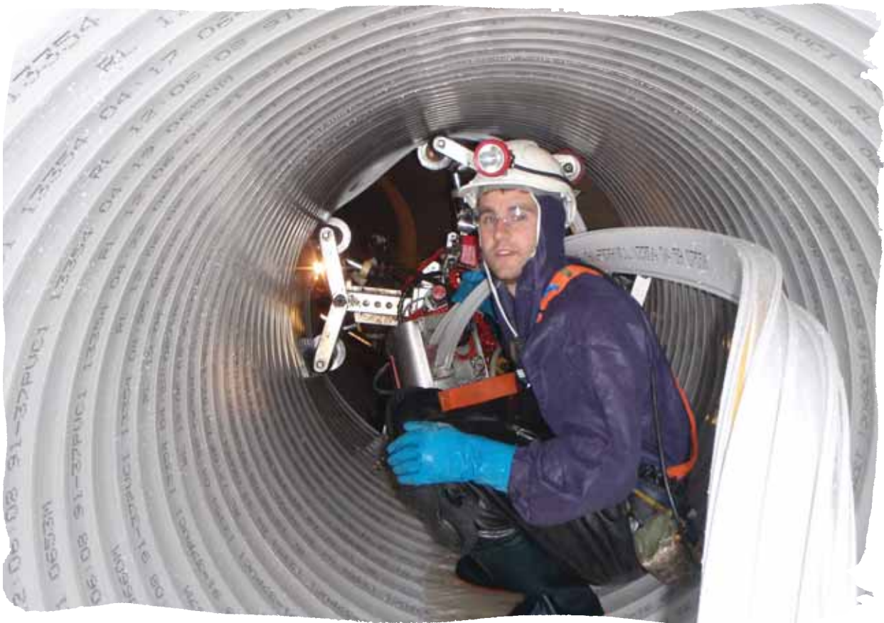
Using a self-winding liner to form a new, stand-alone pipe within a corroded sewer main at Moa Point, near Wellington Airport, saved almost $1 million over conventional replacement methods. Airport disruption was minimised as well.
