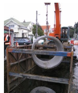
Stormwater pipes put in place in conjunction with the Wellington Inner City Bypass project
