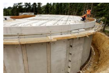
Mt Albert reservoir under construction
