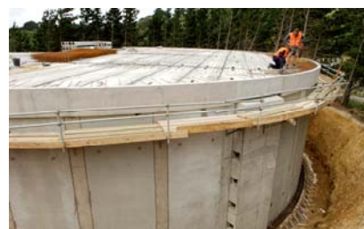
Mt Albert reservoir under construction
