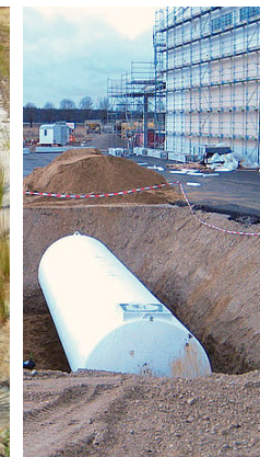
Subsurface rain tank
