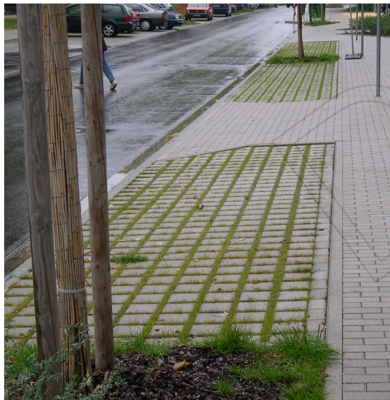
above: example of interlocking concrete block system below example of plastic modular system
