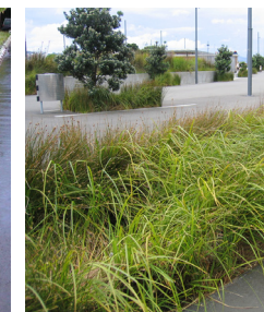
Bio-retention tree pit
