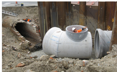
Upgrading the pipe network
