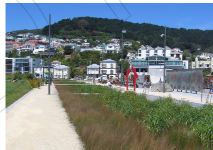
Waitangi Stream has been daylighted in the park, contributing to cleaning the stormwater and creating a strong identity.
