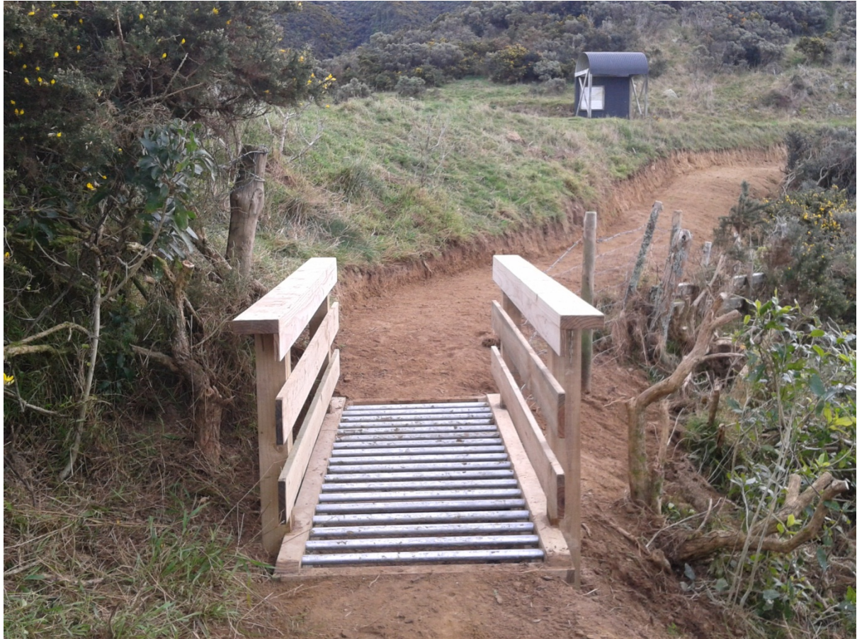
Figure 2. Upper section of track (before the application of gravel) connecting to the ridge leading to the Skyline track. Cattlestop constructed by Kennett Brothers, using WCC resources. Note: the grey lean-to in the foreground was destroyed by storm on 20/6/2013. Image courtesy Simon Kennett.
