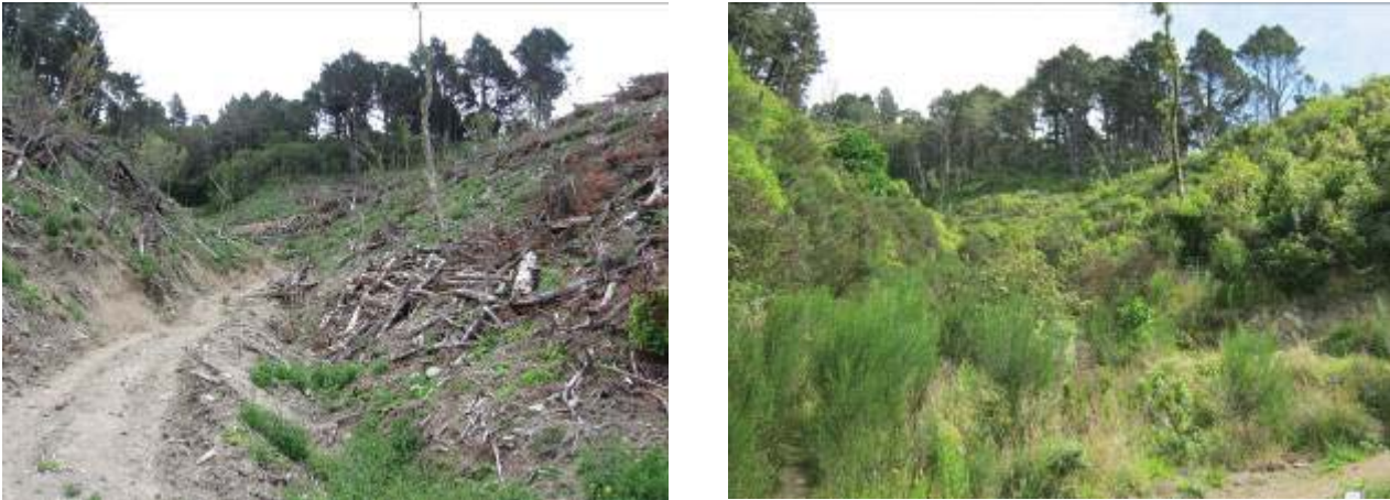
Figure 13: Te Ahumairangi Hill after storm damage in 2004
