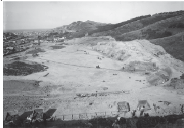
Figure 4: Hataitai Park under construction in 1932. Relief labour dug out banks and moved spoil in metal bins on rails.
