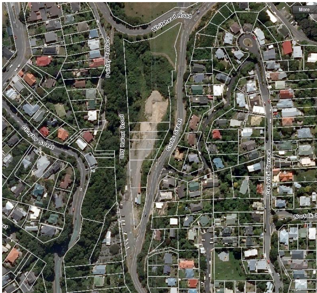
Figure 2: Aerial view of the site, showing vegetation which has developed and formed a canopy over Old Karori Road.
