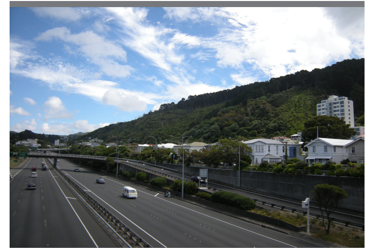
Looking along Tinakori Road from Hobson Street Bridge
