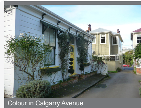
Weatherboards and corrugated iron
