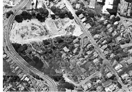
1970 : Aerial showing the beginning of the construction of the motorway.
