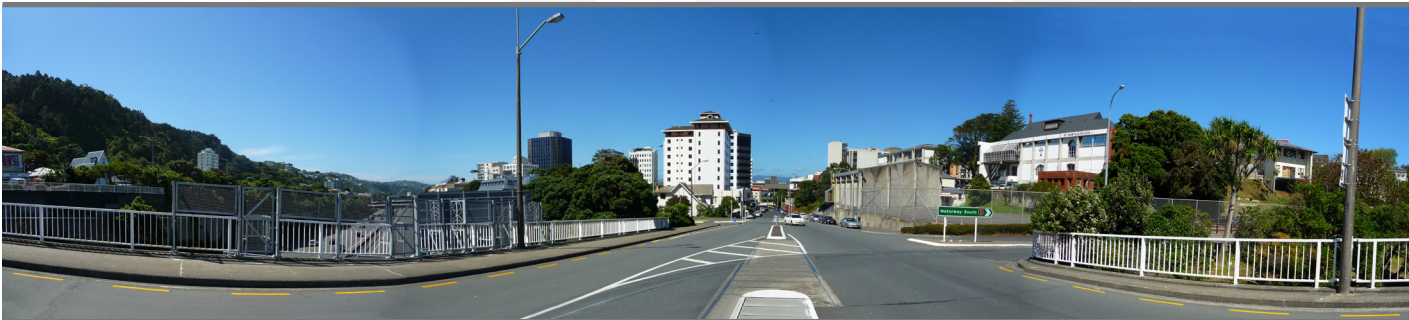
15. Hawkestone Street overbridge
