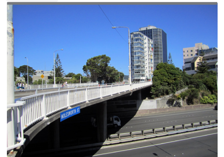
19. Molesworth Street overbridge
