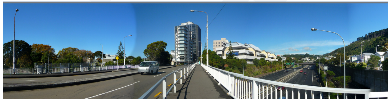
7. The bridge on Molesworth Street over the motorway
