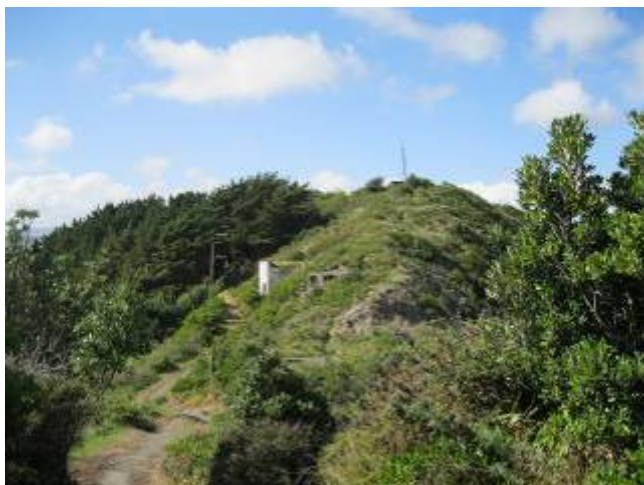
Telecommunications tower on the ridgeline
