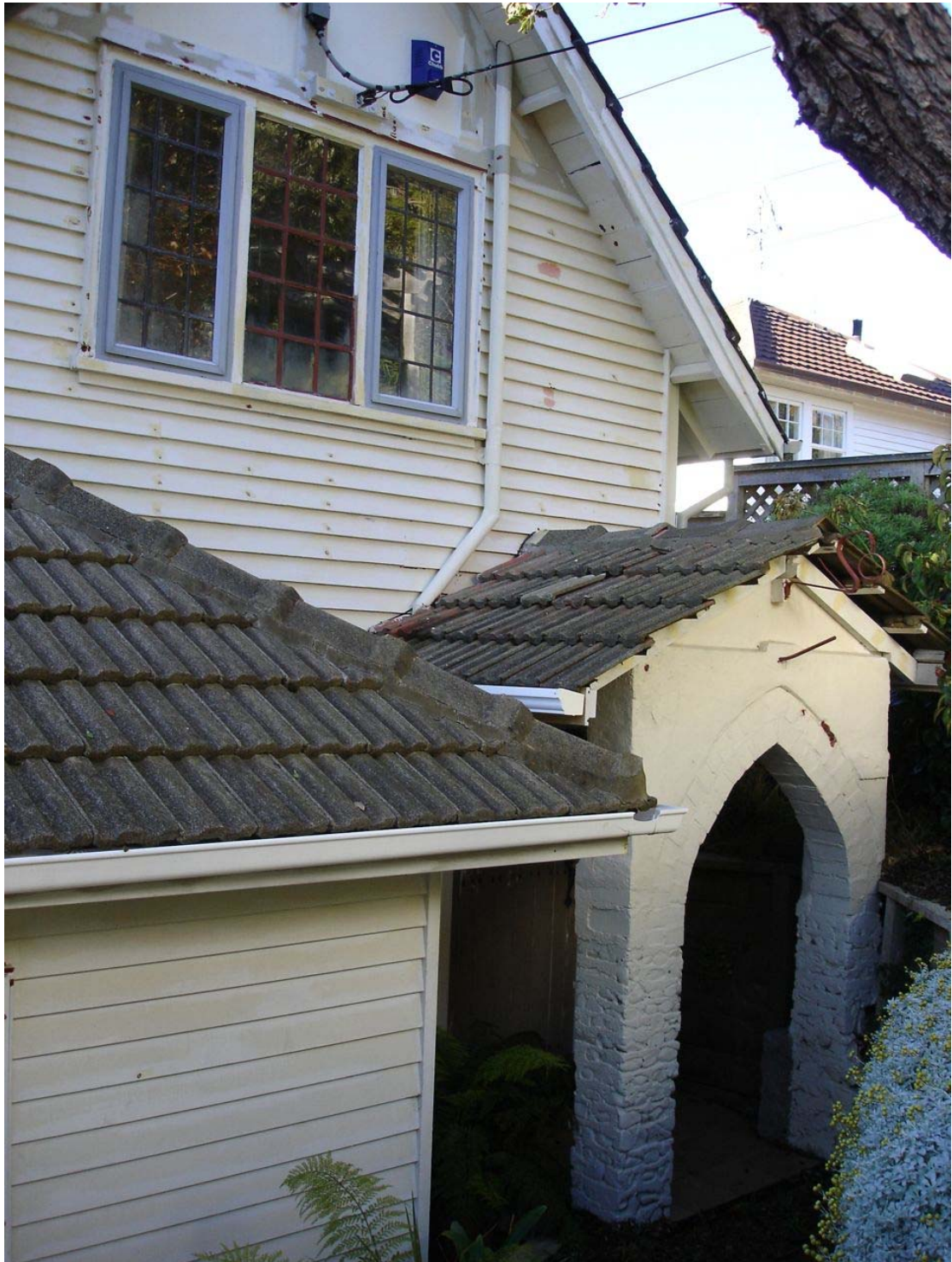
West side - porch addition, kitchen/sun-room extension, replacement windows etc.
