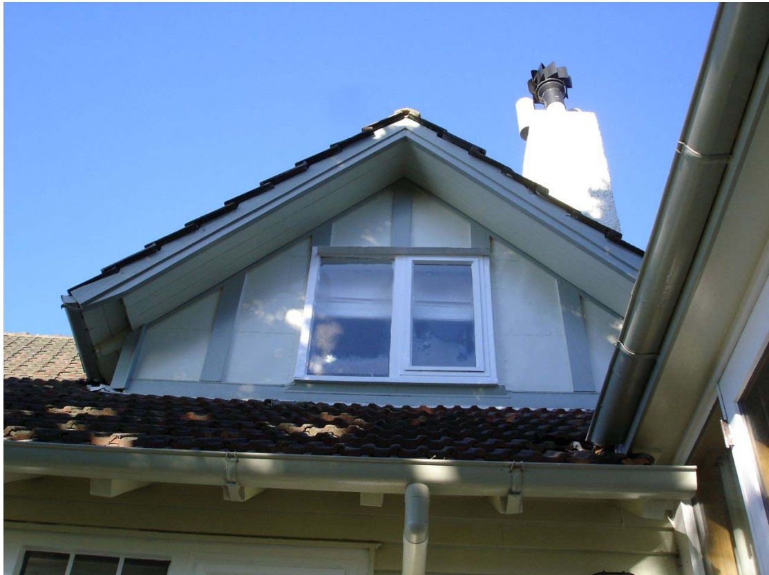
North side - original dormer window and chimney, replacement window joinery.
