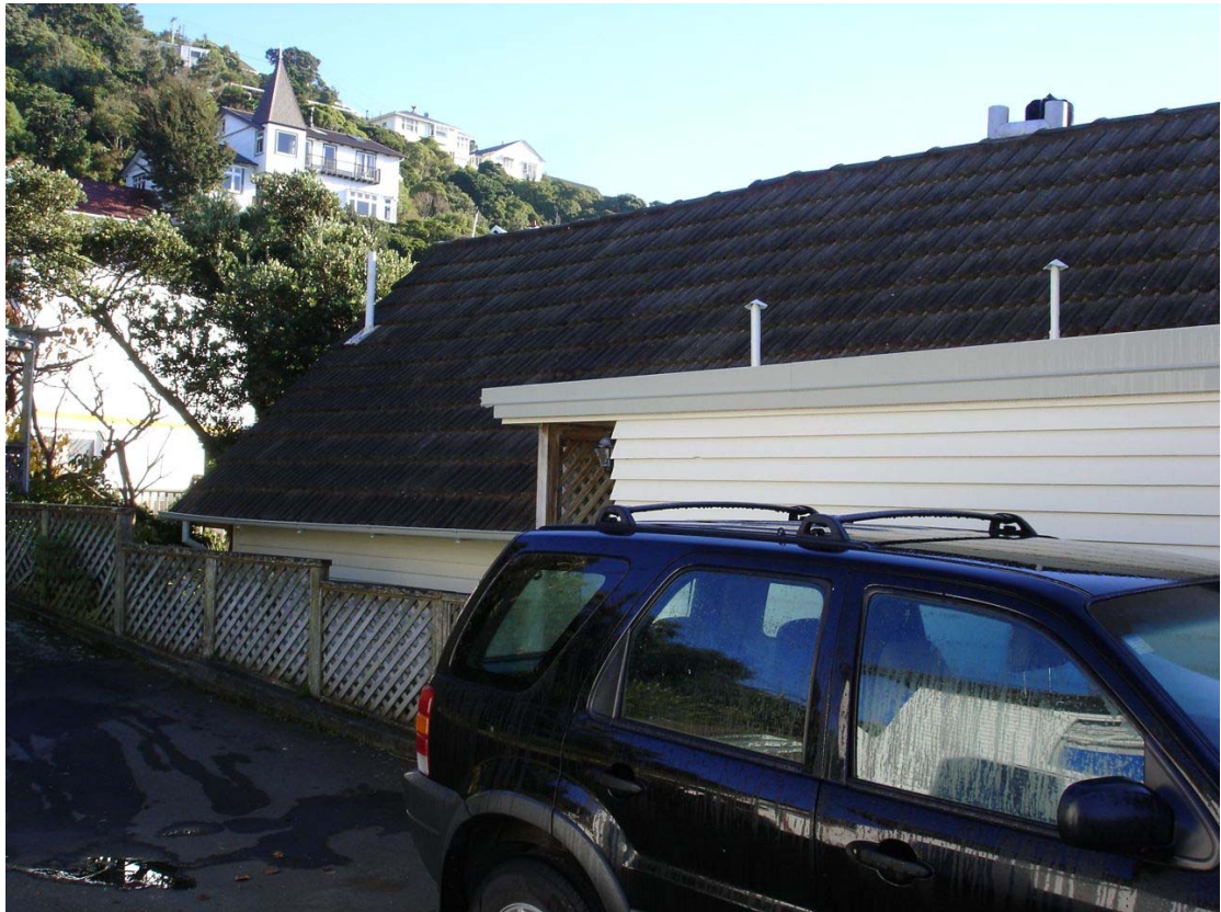
Part of south elevation - bathroom addition prominent in the foreground
