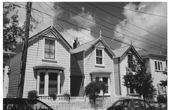
The Cottage is another recurring building type
