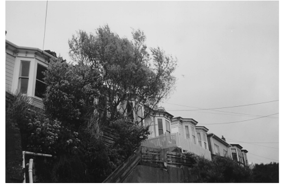
Eastern side of Scarborough Terrace. A notable concentration of identical single villas built over raised platforms.
