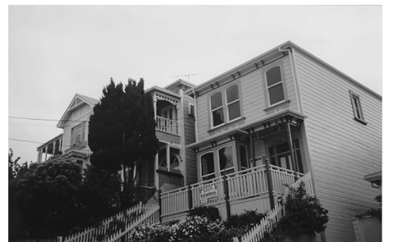
Group of two storey villas in contrast to the predominant setting of single storey dwellings
