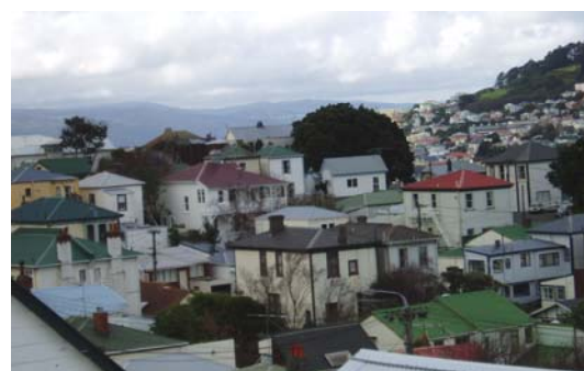
Intricate roofscape demonstrating consistency of roof type and pitch
