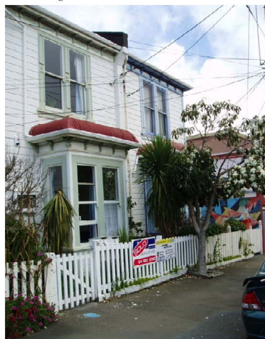
Neighbouring buildings, aligned with each other give a strong street edge definition
