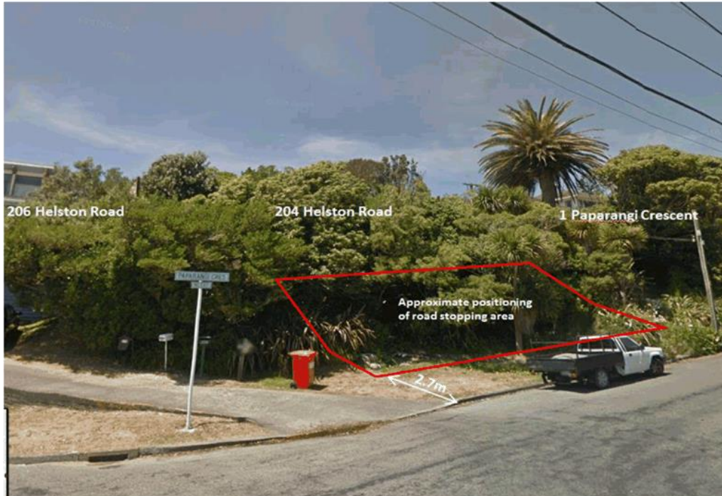
204 Helston Road, Paparangi - views from Paparangi Crescent at street level
