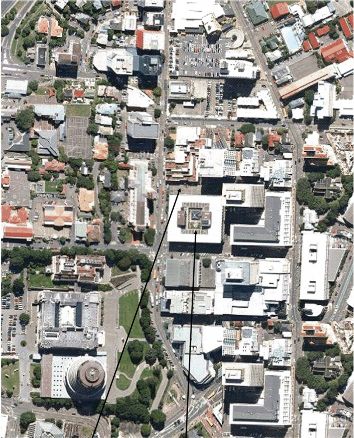
This is where Wingfield St was
