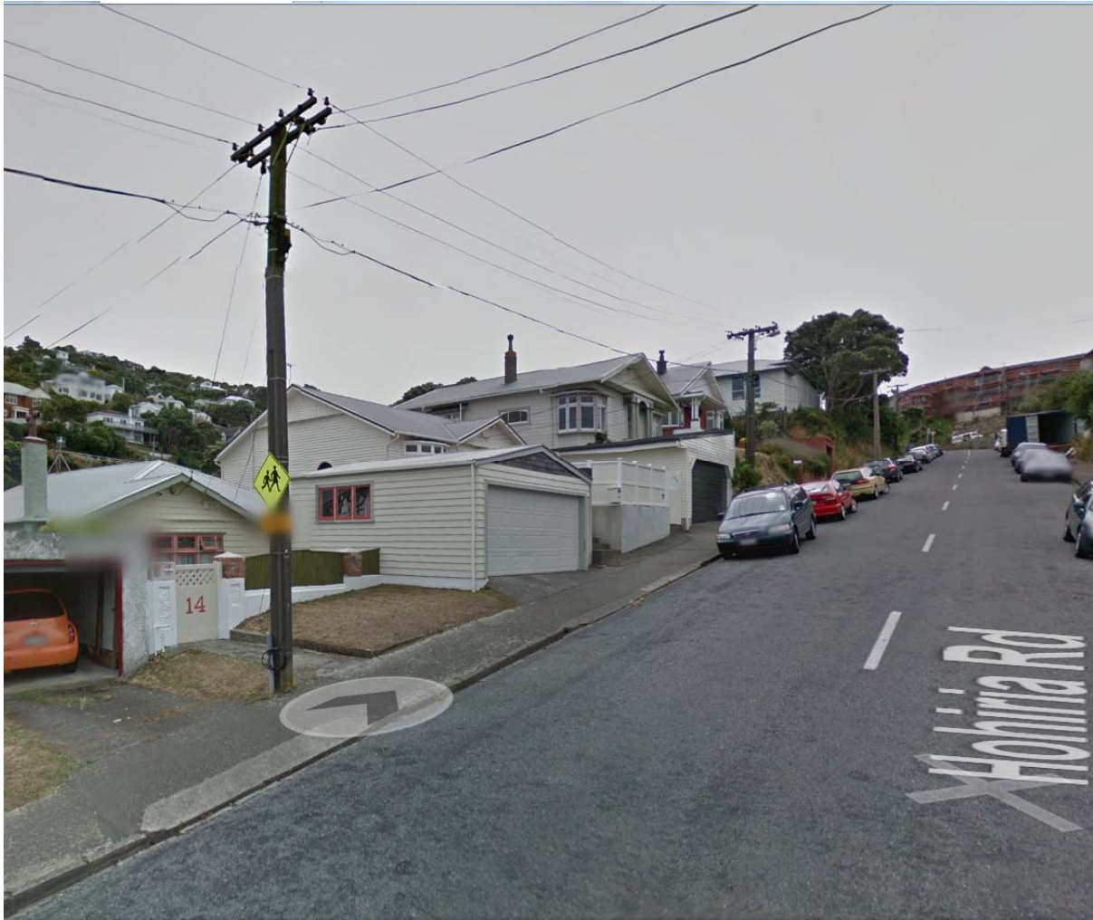
Photo of 12 and 14 Hohiria Road garage and front yard encroachments.
