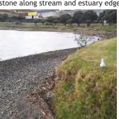
Reclamation material eroded by wave action creates a barrier to water access
