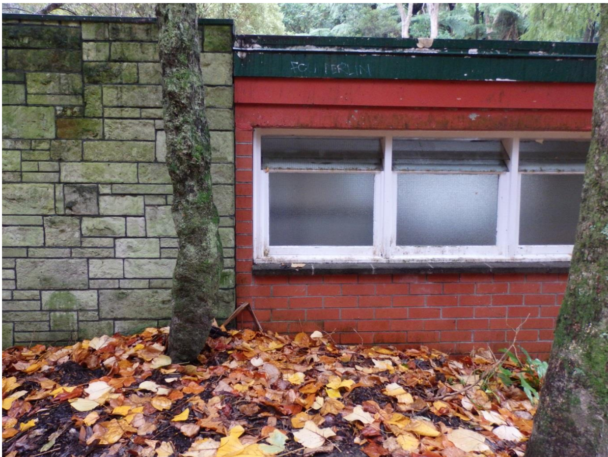
Khandallah pool building, 10 th May 2018. Note dirty peeling paint, moss, mould and mulch.
