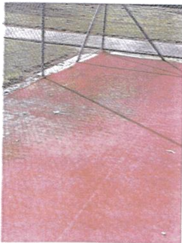
Maintenance is required to keep fibres/infill clean.
