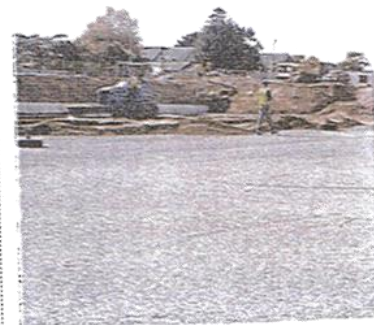
Gravel drainage layer installed and levelled. Sand root-zone starting to be placed.
