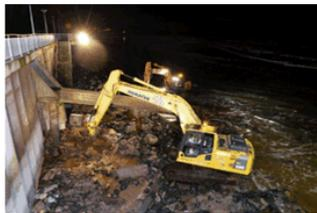
Two diggers begin pushing rock to secure the exposed toe of a concrete panel of the St Clair seawall late last night. Low tide allowed Fulton Hogan contractors to begin work at 10pm, with more work possible at the beach this morning. Photographer not identified [ODT Files]
