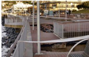
Two large sinkholes created when the Esplanade at St Clair was undermined after the sea gouged a hole under the seawall. Photo: Stephen Jaquierey [ODT Files]
