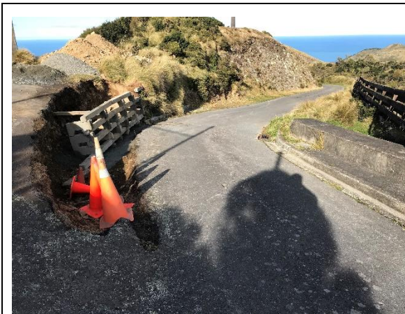
Photograph 3-17: Retaining wall under construction at access to radome
