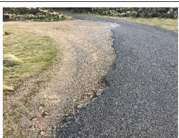
Photograph 3-18: Edge break at start of unsealed RoW section
