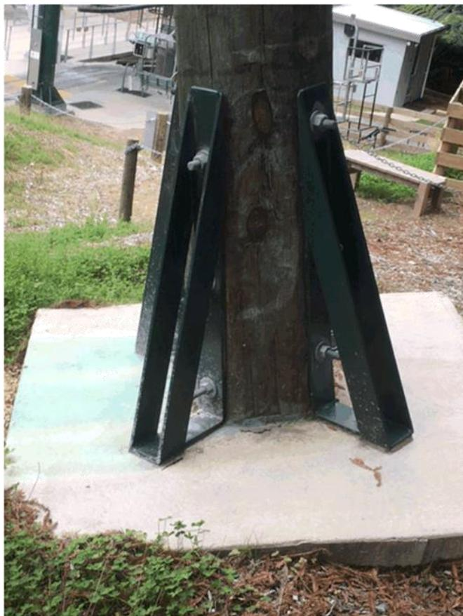
**Figure 14:** Alternate pole footing option. This requires less excavation and soil removal and simply requires a 500mm thick concrete pad to be laid. Note: This is an option for this project but not until proper design projects have been completed would this type of detail be confirmed.
