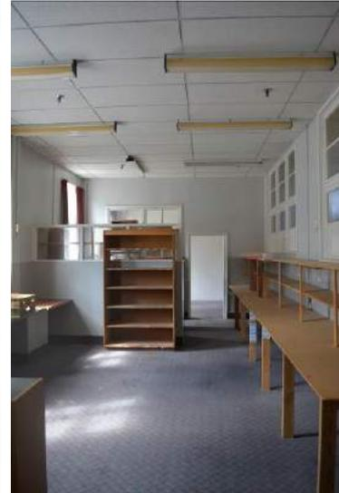
**Fig. 81** View of a typical room in the single storey section of the building. Note the plain sheet linings on walls and ceilings.
