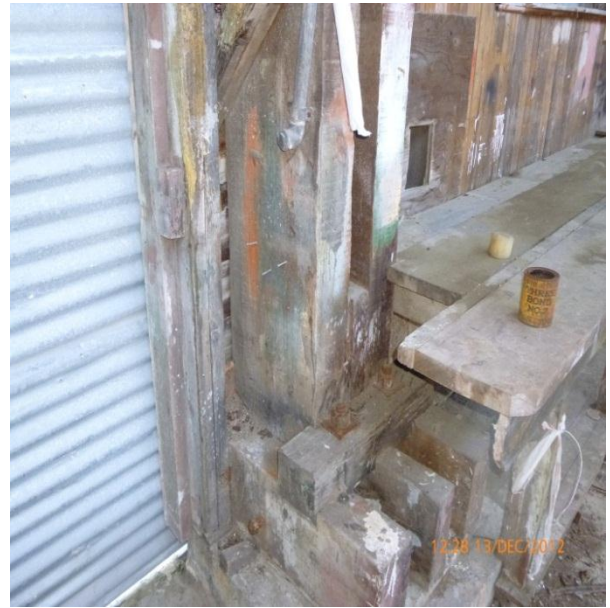
Figure 3: Timber portal column base
