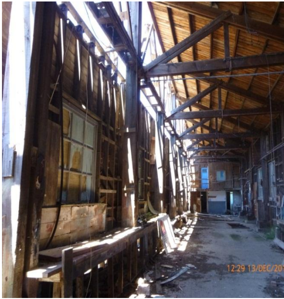
Figure 2: Timber framed external wall
