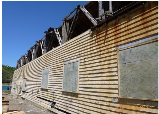
Figure 5: Truss missing top chord members
