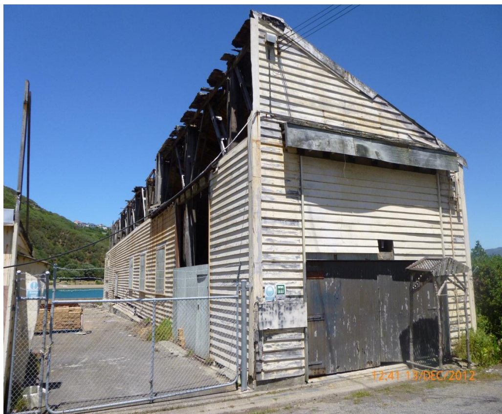
Figure 9: External view of former roller door
