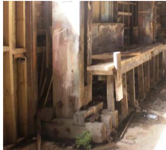
Figure 7: Timber frame base detail
