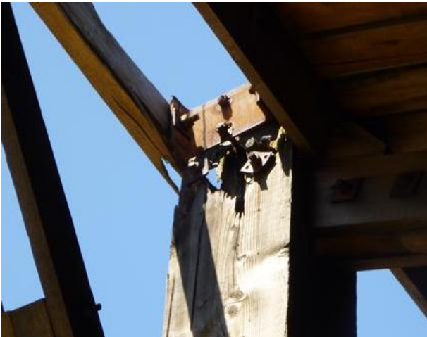
Figure 4: Deteriorated Connection
