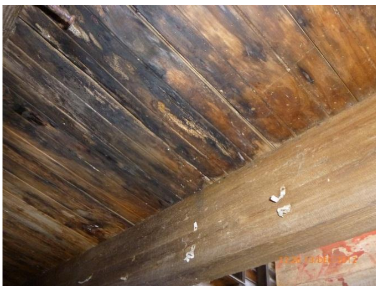
Figure 10: Moisture damage to internal timbers
