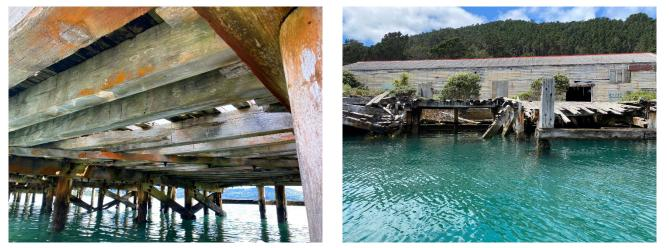
condition of the existing wharf will be formative in the deconstruction methodology. It is assumed generally that no plant, equipment, or materials will be able to access the wharf deck though fear of collapse. It may be possible to complete individual assessments of the structure for access suitability however upon risk assessment we believe that at this stage it is prudent to assume no access is feasible.
