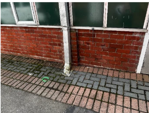
1.29 Spalled bricks in the rear wall veneer
