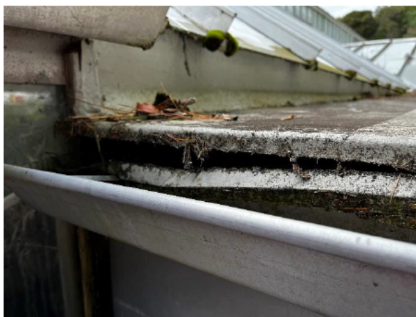
2.10 The drip edge has detached from the roof overhang
