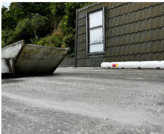
2.7 Link workshop flat roof with membrane lining and liquid plastic overlay
