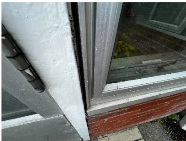
1.19 There is a tapering gap between the door and wall/glazing to the central annex and the cause of the movement is undetermined
