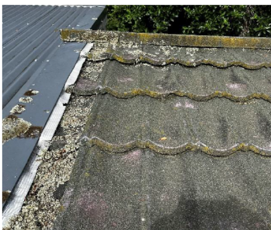
2.19 The roof junction flashing is poorly installed
