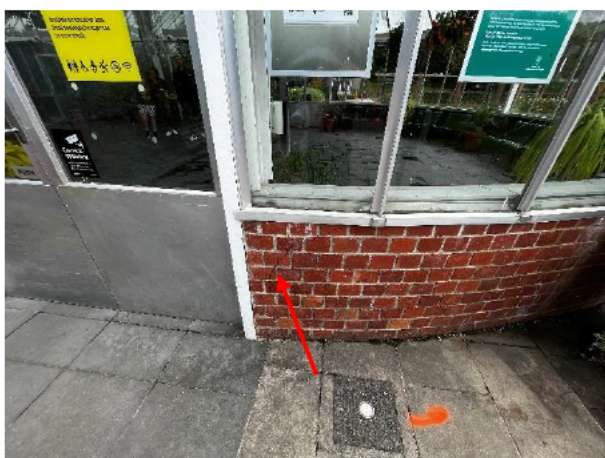
1.19 There is a tapering gap between the door and wall/glazing to the central annex and the cause of the movement is undetermined
