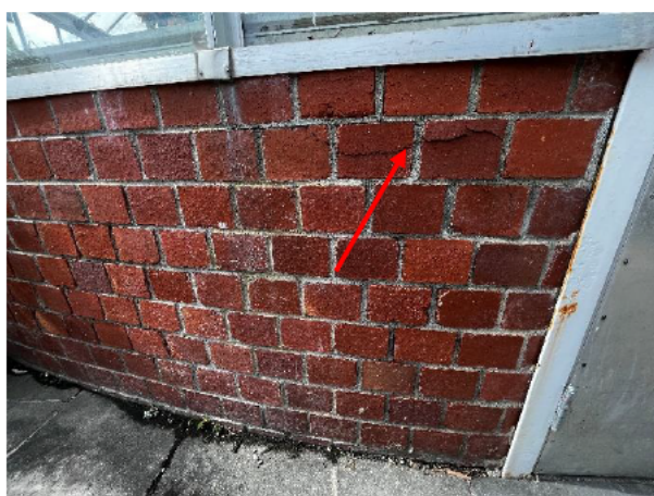
1.18 Damaged bricks located on the west elevation next to the door on the central annex
