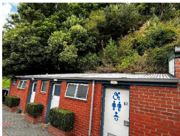
2.22 Toilet block roof cladding has attained the end of its design life and is recommended for replacement
