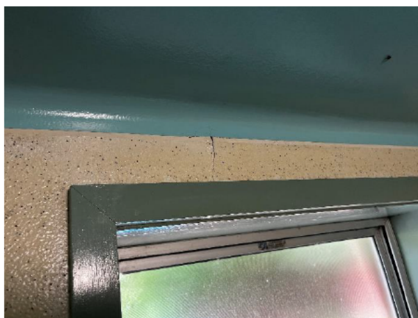
1.110 Cracked wall board joint with moisture damage
