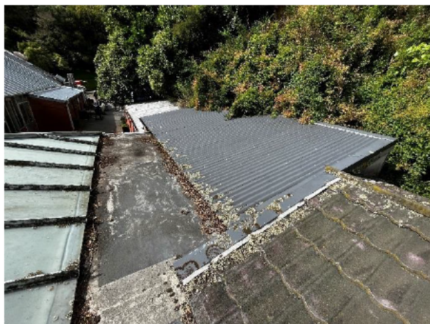
2.18 Roof cladding reward of the central annex has recently been replaced. The flat roof membrane is perished and requires replacement
