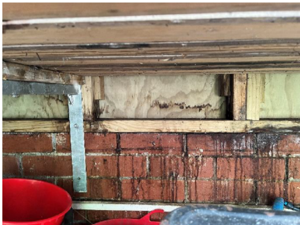
1.95 Moisture damaged wall framing and substrate in the potting shed
