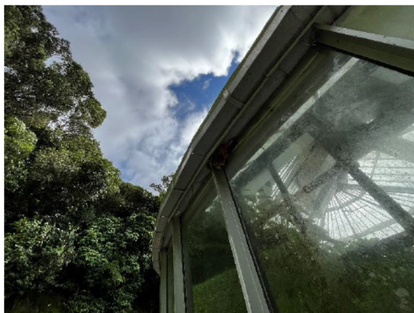
1.152 Open gutter joints
