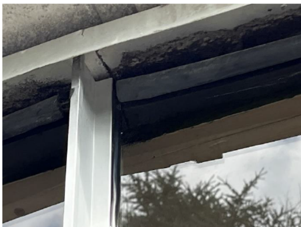
1.79 Internal gaskets have dropped
