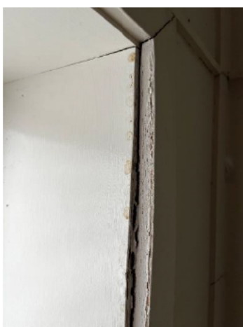
2.54 Rear office moisture damaged window trims and frame
