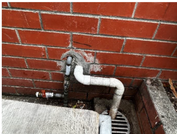
1.26 Example of unsealed penetrations through the veneer
