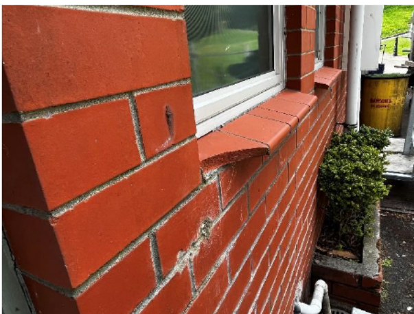
1.27 Damaged sill and unsealed penetration
