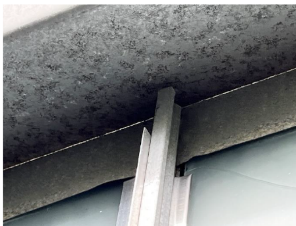
1.58 Glazing bead cut short
