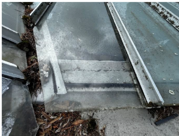
1.36 Corner junction is leaking into the roof frame below
