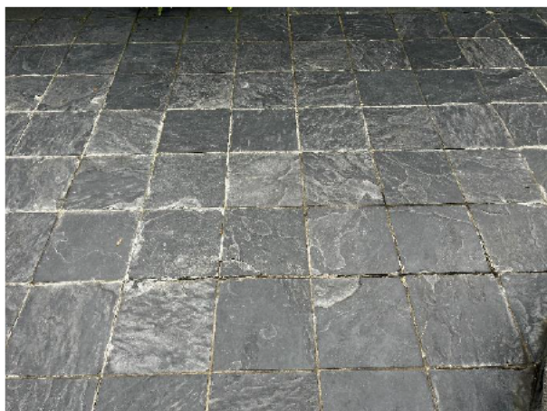
1.113 Delaminating floor tiles
