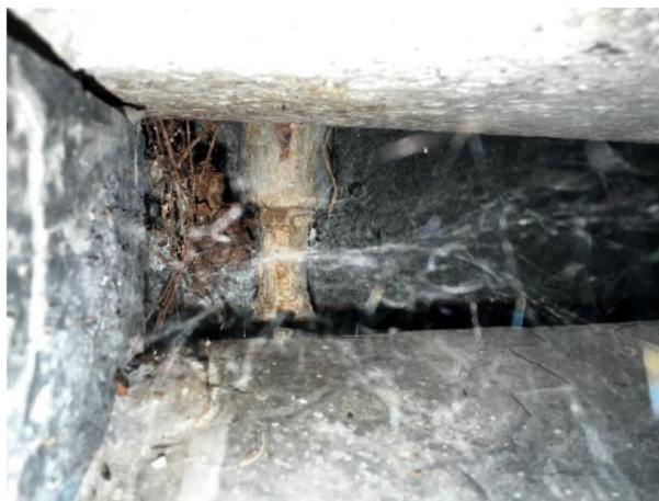
1.138 Heating pipe branch in temperate zone
