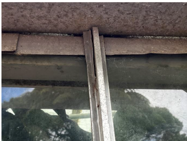
1.49 Aluminium, glazing bead is split and dislodged
