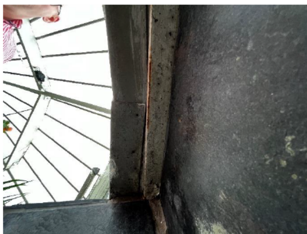
1.10 Isolated surface corrosion on a perimeter beam
