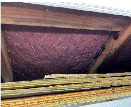
2.13 Decayed roof framing
