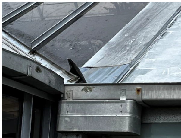
1.62 Flashing has deflected and lifted on the bottom corner junction with the cafe
