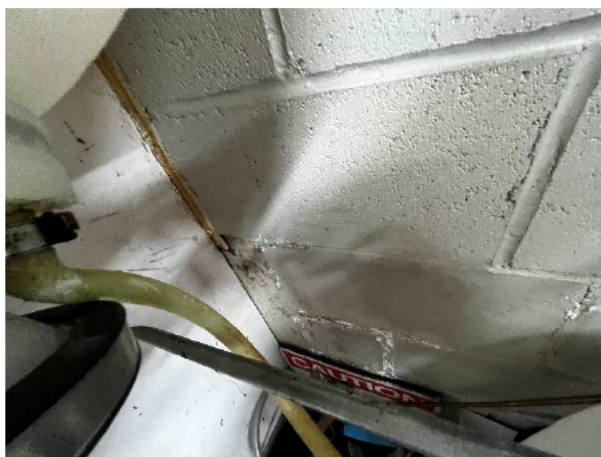
2.39 The corner wall junction has been infilled with expanding foam to create a weatherproof seal. Efflorescence and moisture staining was observed
