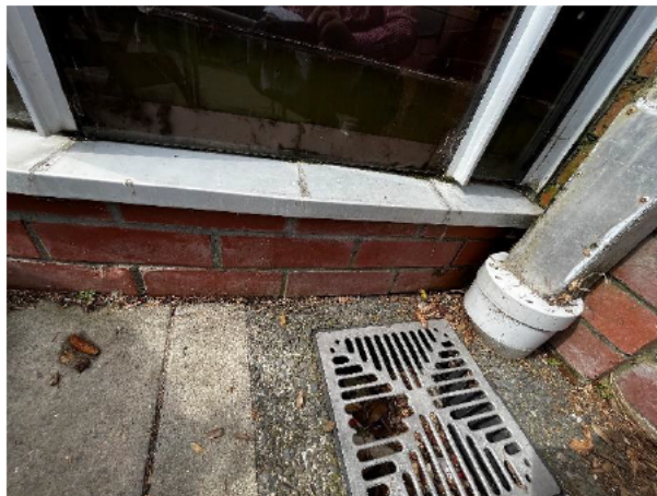
1.66 Poorly sealed junction between the wall and glazing system creating a moisture ingress route
