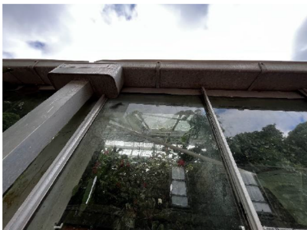
1.151 Gutter fixings are corroded
