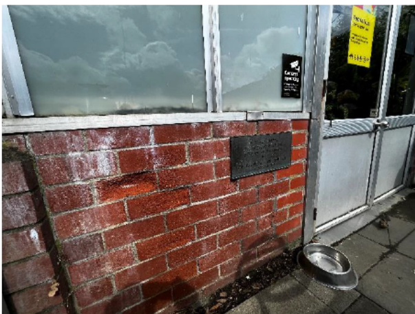
1.25 Spalled and degraded bricks to the door panel of the east annex note that the plaque states that the tea house was constructed circa 1981 and the joinery is therefore at end of life.
