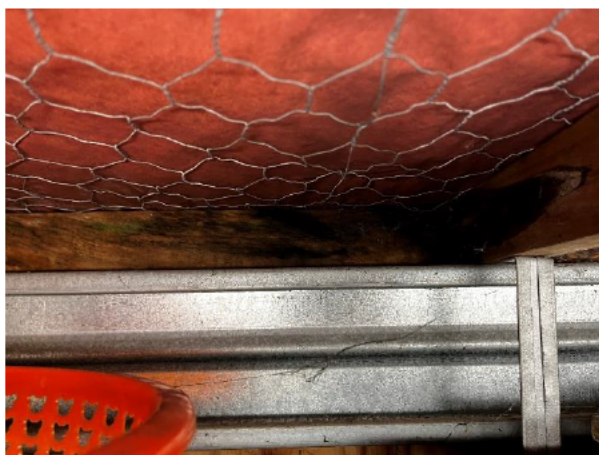
2.16 Decayed roof framing
