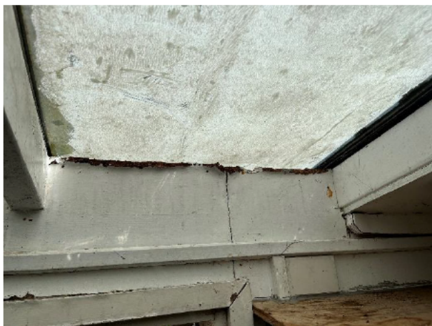
1.91 Internal damage to the potting shed skylight walls
