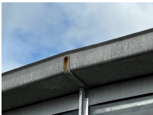
1.154 Corroded gutter brackets
