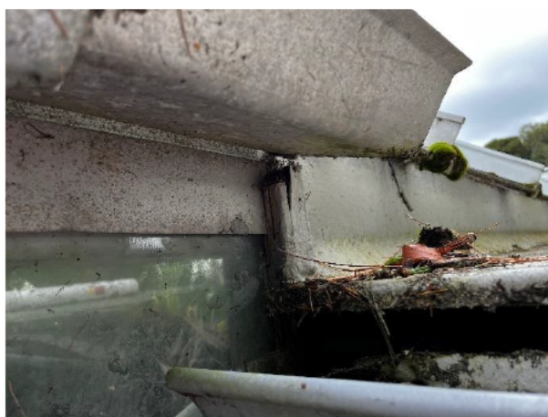
1.40 The link extension is incorrectly built into the glass house creating moisture ingress routes and damage
