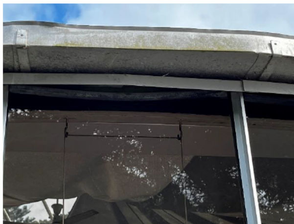
1.80 Gaskets have worked loose
