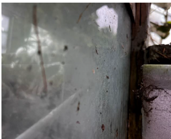
2.9 Unsealed junction between the glasshouse and workshop fascia's
