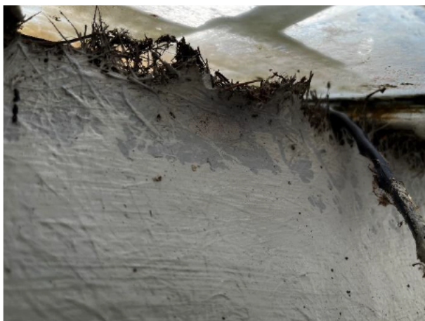
1.85 Gaskets have fallen out and condensation from the glasshouse roof is running into the wall frame
