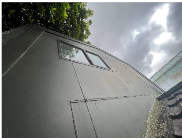
2.27 Popped nail fixings, cracked boards, and damaged jointing strips
