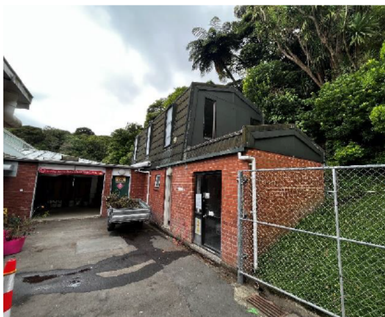
2.34 The building is set into the hillside and the gable and rear wall does not appear to have been adequately waterproofed, if at all
