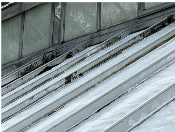
1.51 Glazing beads are missing leaving one side of the glass panel insecure and the glazing panes are delaminating
