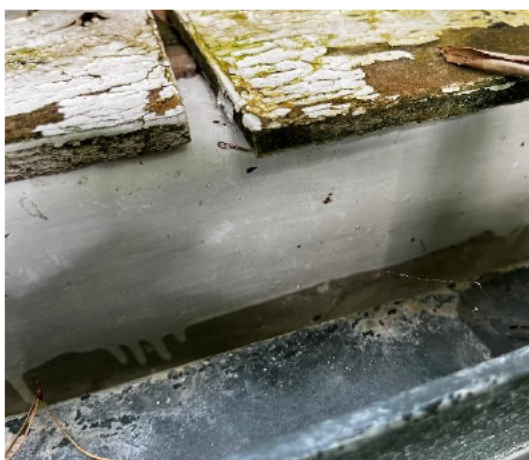
3.9 Internal windows sills are moisture damaged
