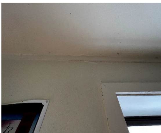
2.30 The wall to ceiling junction is moisture damaged and staff informed that water penetrates when the wind blows from a norther direction
