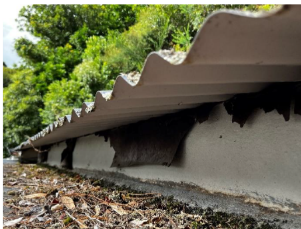
2.18 Roof cladding reward of the central annex has recently been replaced. The flat roof membrane is perished and requires replacement
