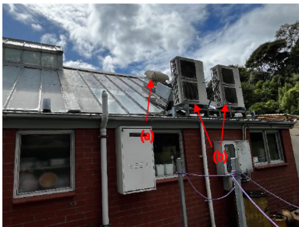
1.141 The (a) extract fans and (b) air conditioning pumps are at the end of economic life.
