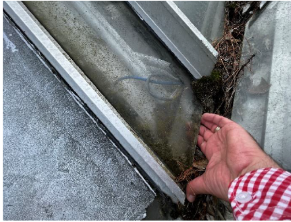
1.78 Gasket missing to base of glazing pane
