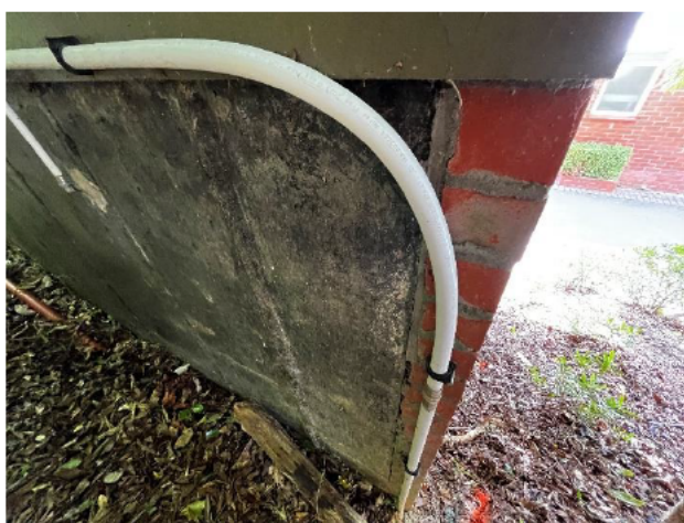
2.43 The gable to rear wall junction is missing mortar and appears to have been incorrectly waterproofed creating a moisture ingress route into the wall frame
