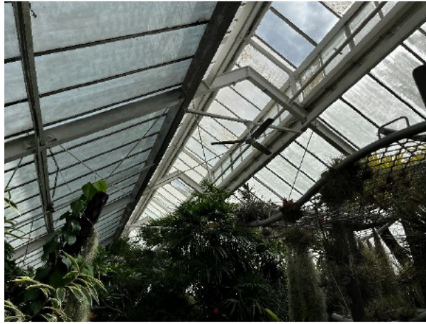
1.142 Air circulation fans are at the end of their design life
