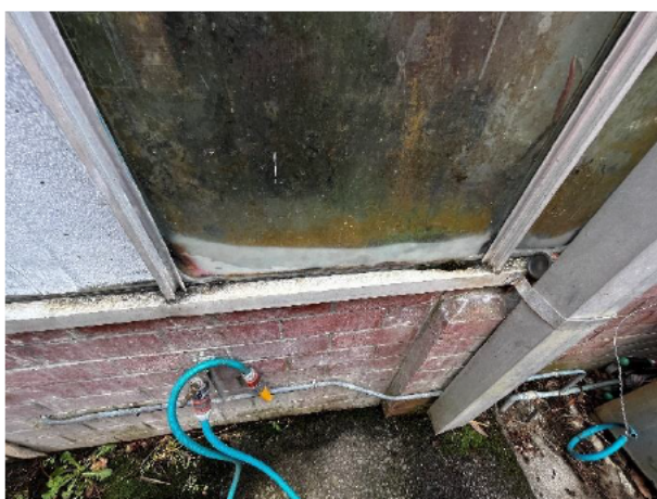
1.75 Delaminating pane
