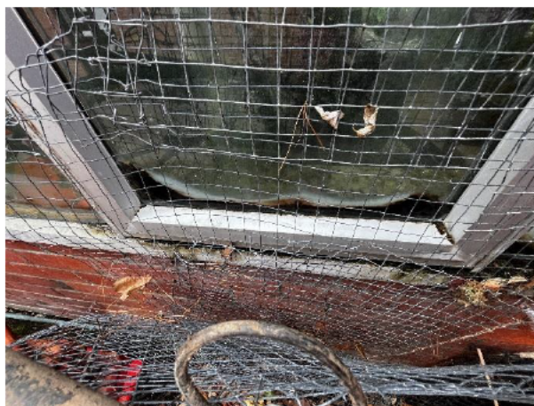
1.46 Open mitre joints and corrosion
