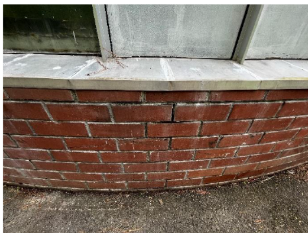
1.16 Cracking in the mortar joints located on the west elevation
