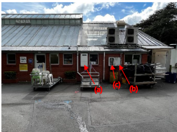
1.125 Rear kitchen and toilets showing (a) hot water boiler and (b) electrical distribution board and (c) meter for the kitchens.
