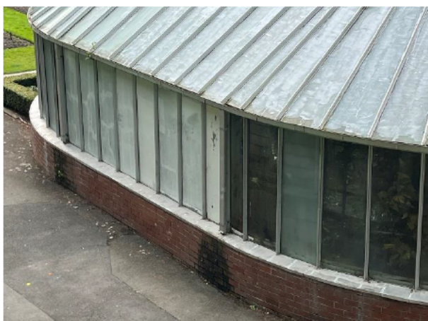
1.149 Gutter joints have failed
