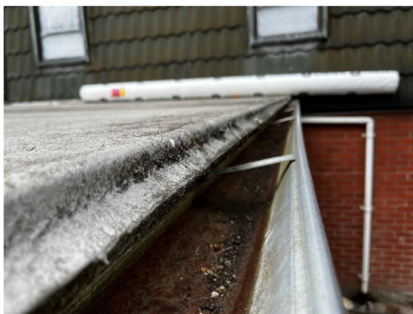
2.8 Gutters are corroded
