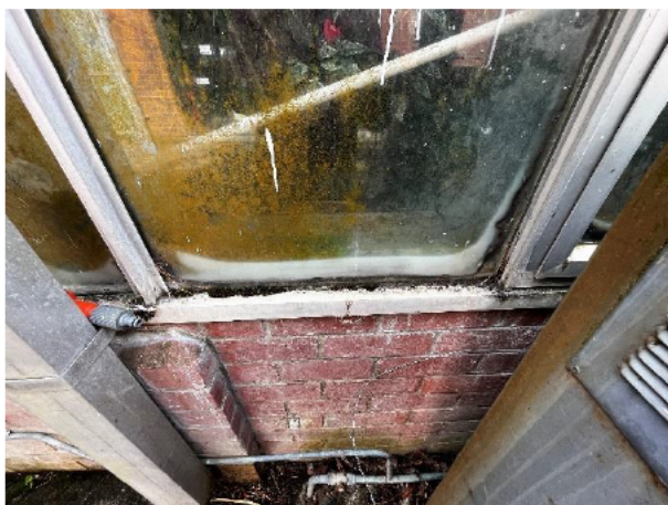
1.49 Aluminium, glazing bead is split and dislodged
