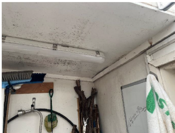
1.92 Mould on the potting shed ceiling and moisture damaged cornice
