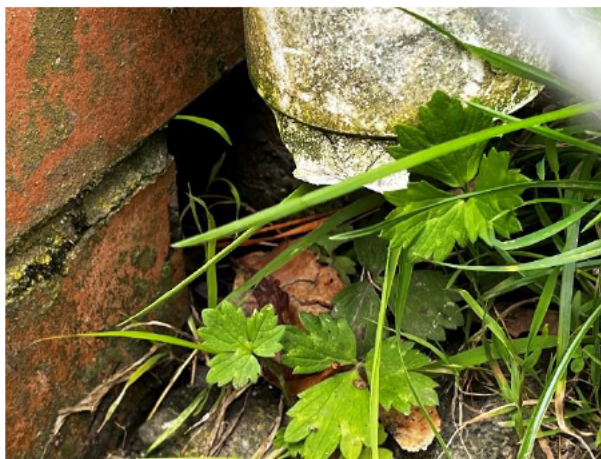
2.35 Hole in the brick veneer where the downpipe terminates
