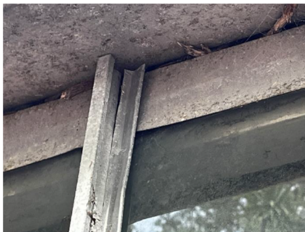
1.50 Aluminium, glazing bead is split and dislodged
