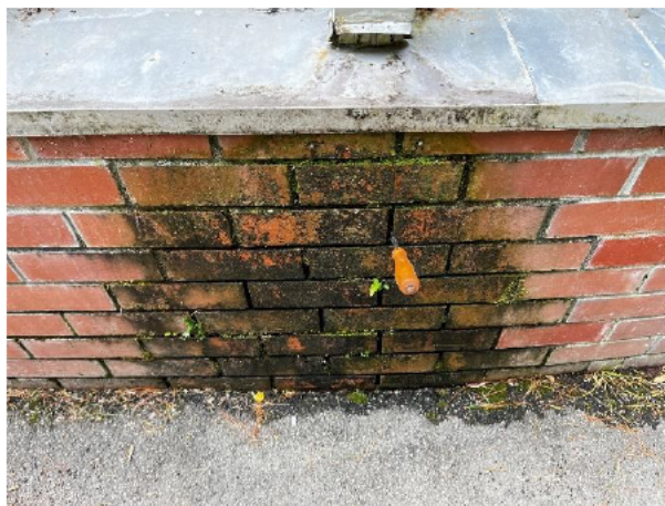
1.32 Mortar joints have degraded where the downpipes terminate.
