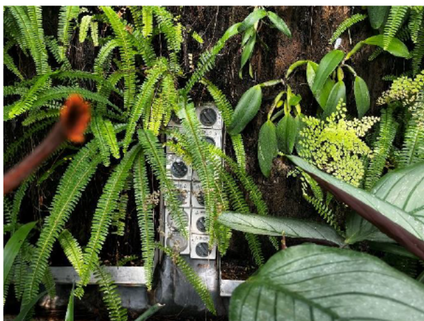
1.121 Electric switch array is constantly wet?
