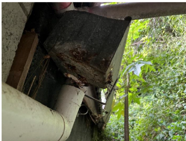
2.24 Rear gutters are corroded
