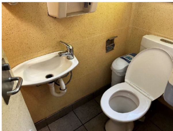
1.108 The sanitary ware is operable. The linings are dated and worn
