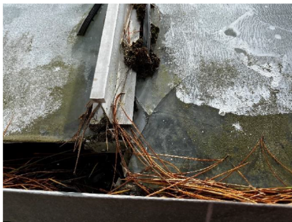
1.84 Slipped and dislodged pane and gaskets
