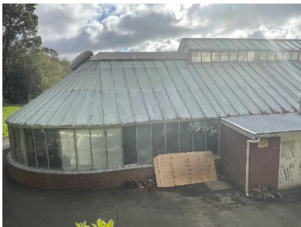
1.73 The glazing panels are whitewashed which requires regular high cost maintenance
