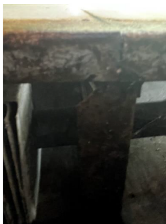
1.134 Framework is corroding around the radiator covers
