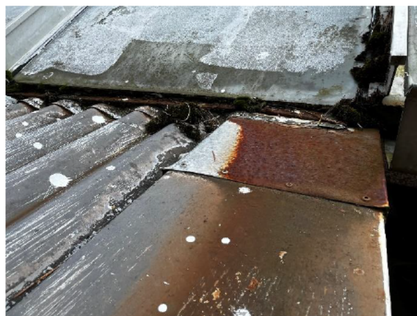
1.88 Corroded barge caps and apron flashings
