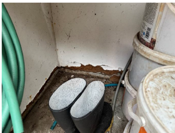
1.94 Moisture damage to the bottom edge of the wall linings
