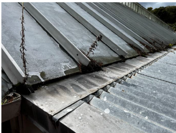
1.83 Slipped gaskets and vegetation growth through deferred maintenance
