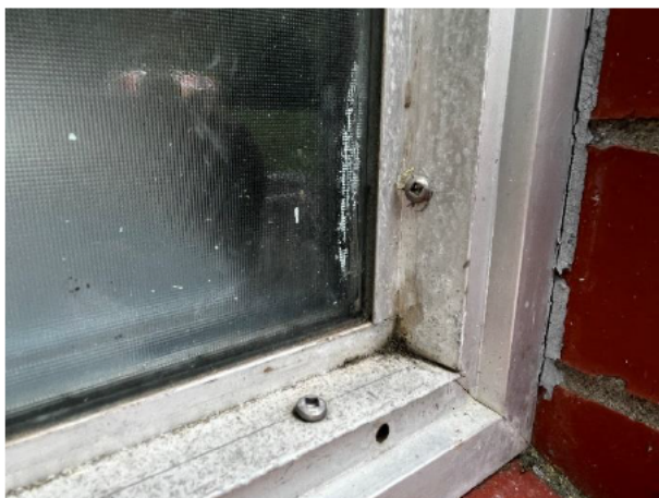
1.102 Windows are fastened shut and the perimeter sealant has failed
