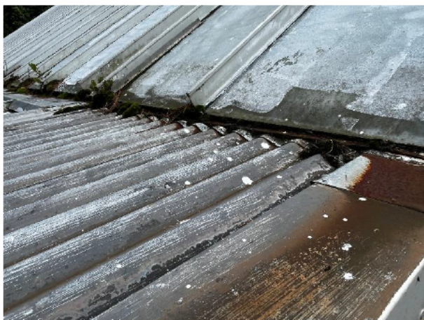
1.89 Corroding edges to roof sheets and vegetation growth
