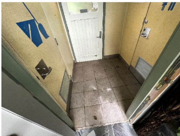
1.107 The toilet entrance wall, floor and ceiling linings and tiles are beyond economic life
