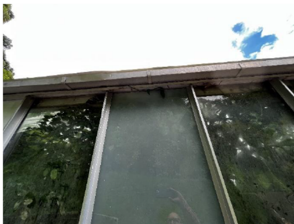
1.54 Plants growing through between the glass and frame
