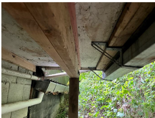
2.37 Rear wall junctions appear to have been poorly detailed
