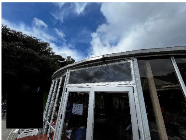
1.155 Defective gutter joints
