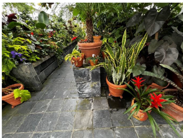
1.114 Floor and planter box tiles are lifting in isolated area, are chipped throughout but remain serviceable though are becoming dated and unsightly
