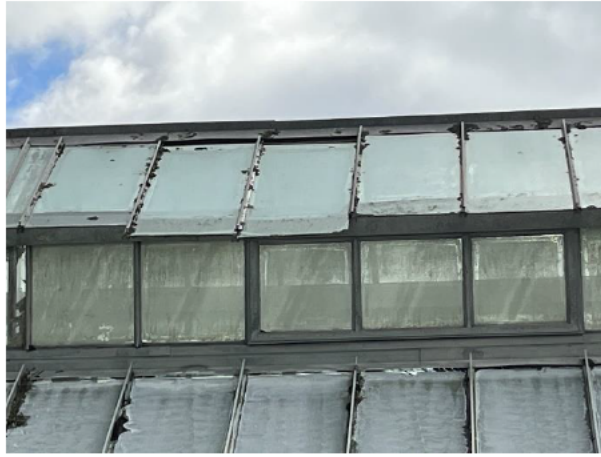
1.72 Slipped panes on the lantern
