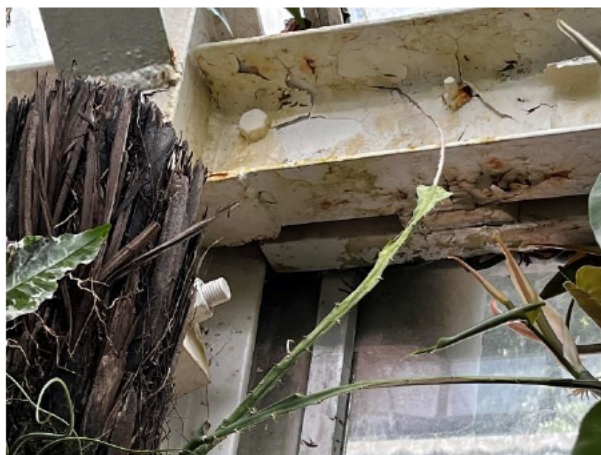
1.4 Corroded beam and damaged painted finish
