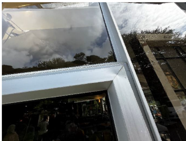
1.68 Open and damaged mitre joint both sides
