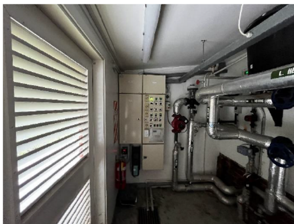
1.124 Electrical switch gear we understand is circa 1988-1991. The heating and hot water supply pipework appears to be in moderate condition within the boiler room. WT understand the main electrical supply cable was replaced in 2021
