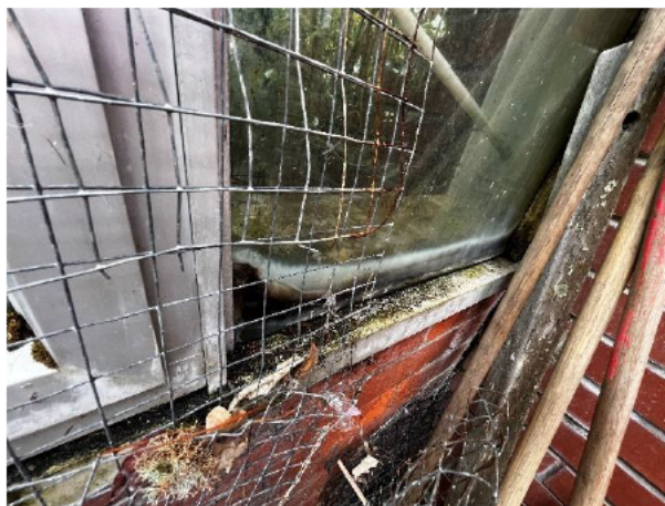
1.74 Bottom edges of the laminated glass panel are delaminating
