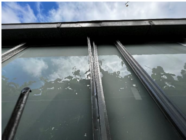
1.59 Glazing bead damaged and detached
