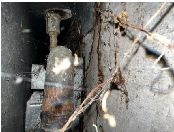
1.137 Pipework and branch from the heating pipes in the temperate zone
