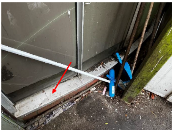
1.67 Impact damage to the window frame
