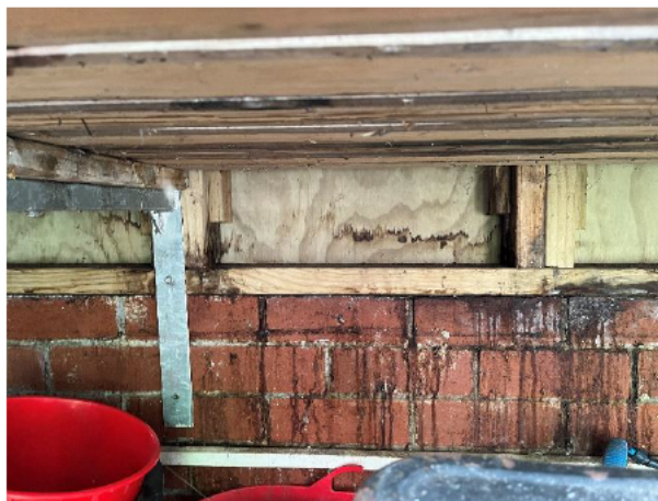
1.34 Moisture damaged timber frame and plywood substrate below the potting shed bench
