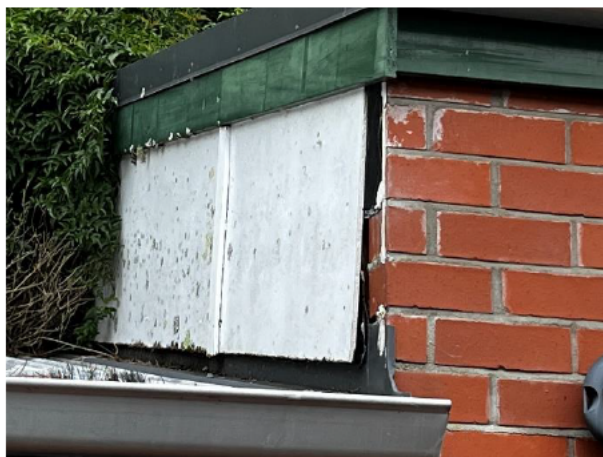
2.33 Direct fixed wall cladding has detached and created a water ingress route into the roof and walls
