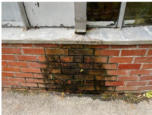
1.56 Downpipe cut short assume because the bottom section damaged by vehicles. Result is damage to the wall.
