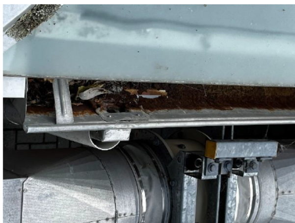
1.150 Gutters corroded through
