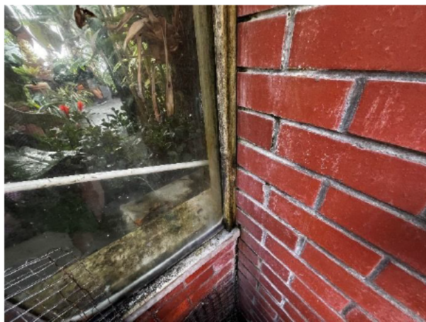
1.48 This junction no longer performs a weathertight seal
