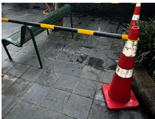
3.6 All loose floor tiles to be lifted and relayed or replaced
