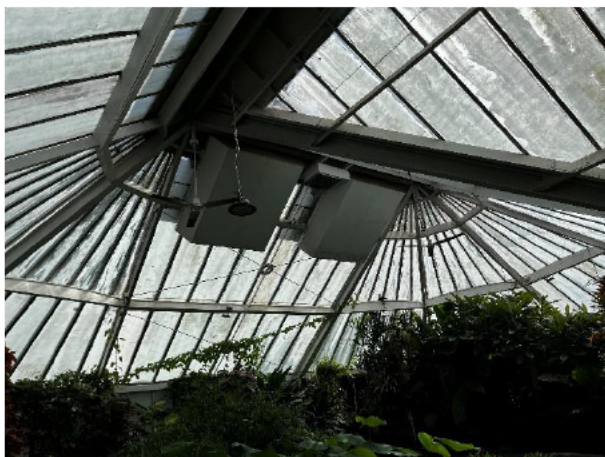
1.143 Air extraction units are at end of life
