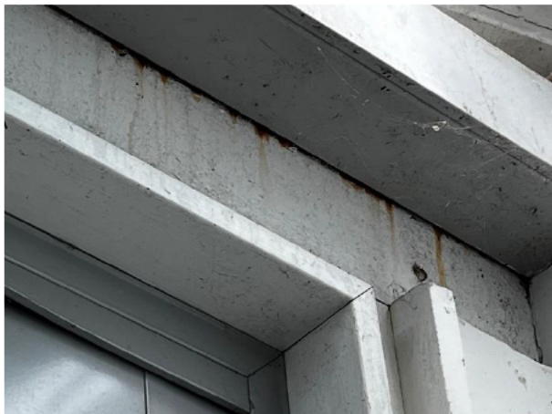
1.11 Corrosion in the lintol above the doors to the central annex back of house
