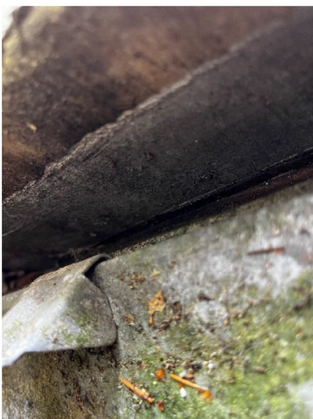
2.11 Roof framing has darkened and appears decayed
