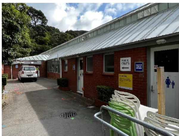
1.101 Door joinery to the toilets is in moderate condition but the aluminium joinery units are in poor condition.,
