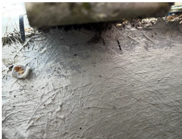
1.44 Unsealed bottom edges of the glazing panels
