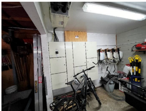
2.65 New distribution boards and supply
