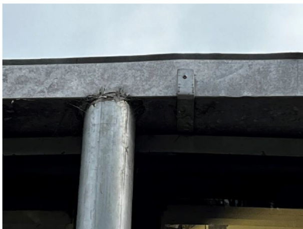
1.157 Corroded outlet
