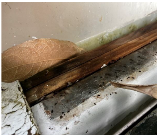
3.7 Timber framing below the sills is moisture stained
