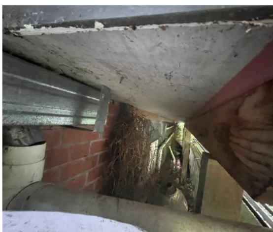
2.44 Rear retaining brick and concrete wall junctions are poorly waterproofed resulting in moisture ingress
