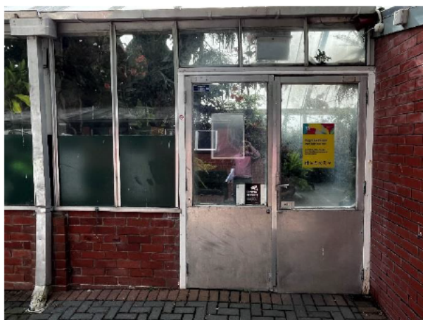
1.97 Doors are out of alignment and corrosion in the frame
