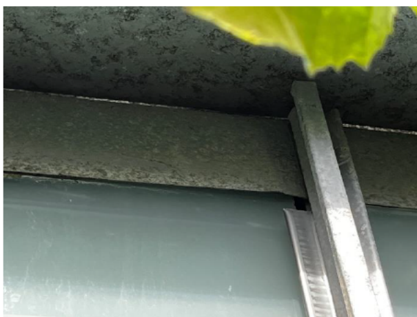
1.57 Glazing beads cut short or slipped
