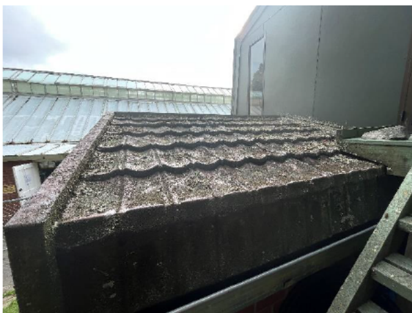
2.2 Dry room roof is deflected and worn. Presumed ACM.
