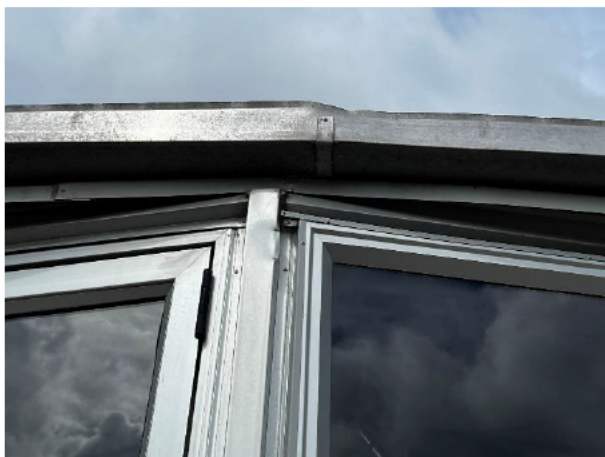
1.67 Impact damage to the window frame
