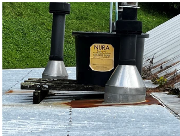
1.90 Corroded back flashings
