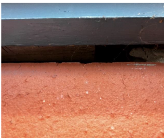
2.19 The roof junction flashing is poorly installed
