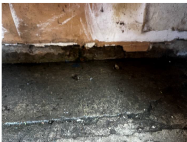
2.47 The dry room floor is saturated from external moisture engrossing into the dry side of the wall
