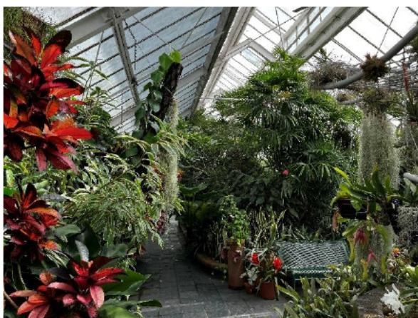
1.1 View from inside the tropical zone showing the steel portal frame, roof purlins and the lantern skylight
