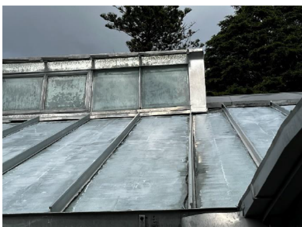
1.41 Apron flashings to the lantern have lifted
