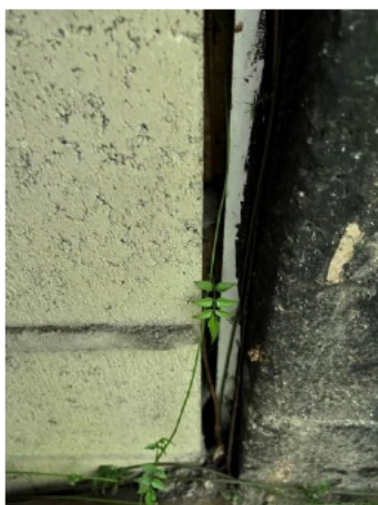
2.38 The junction is packed with timber and expanding foam
