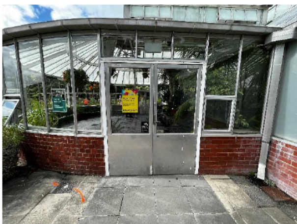
1.98 Defective and damaged doors with corrosion in the steel frame
