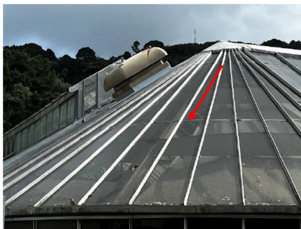
1.70 Glazing joint sealant has failed resulting in damage to the kitchen ceiling
