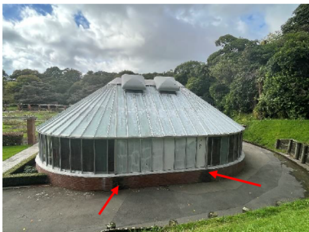
1.31 West annex. Arrows indicate where the gutter downpipes drain onto the perimeter wall
