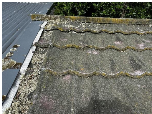
3.1 The coating of Decramastic tiles is known to contain asbestos
