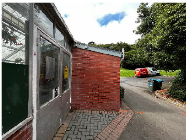
1.96 These double door joinery units are at end of life and recommended for replacement. The steel perimeter frames are corroded and either require repair or replacement
