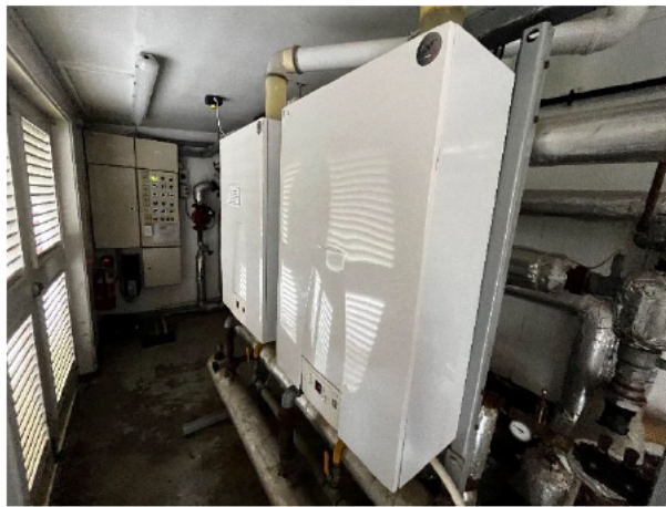
1.140 Condensing boilers are 10-12 years old and remain in an operable condition but are nearing end of economic life.
