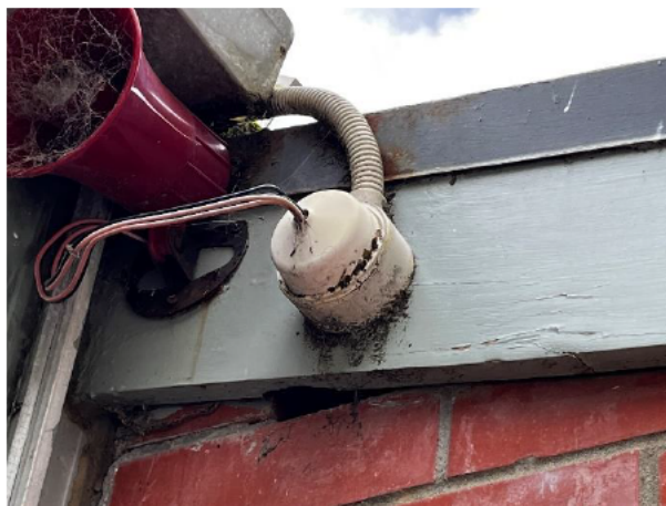
1.28 Gap between the barge and wall veneer creating a vermin access point
