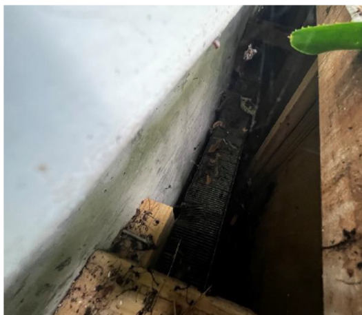
3.8 Mock timber wall is water damaged
