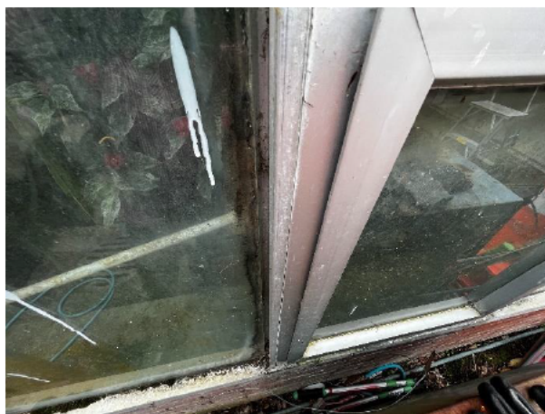
1.52 Missing glazing bead
