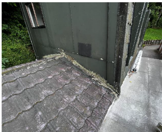
2.26 Direct fixed external wall cladding system is defective and damaged
