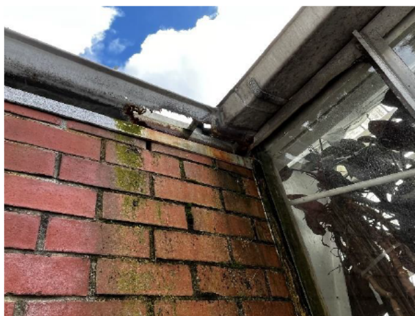
1.30 Gap between the link wall and glass house creating a water access route into the wall frame.
