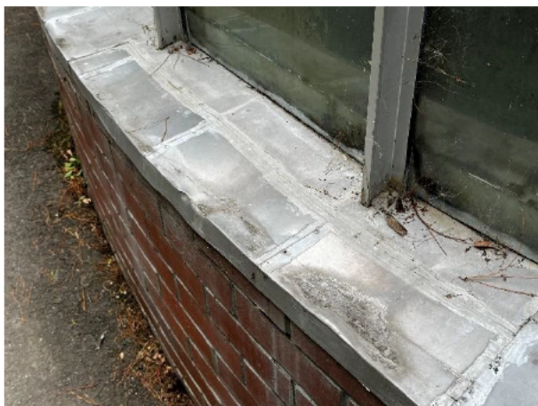
1.55 Damaged and poorly repaired sill
