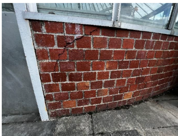
1.22 Close up view of the cracked veneer
