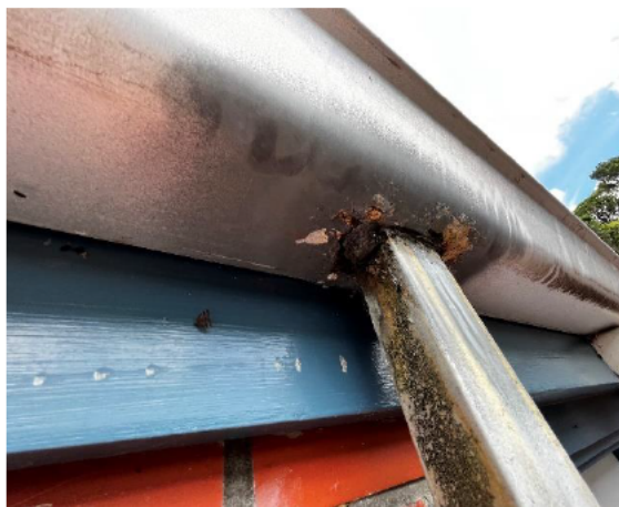
2.23 Gutter outlet is corroded through
