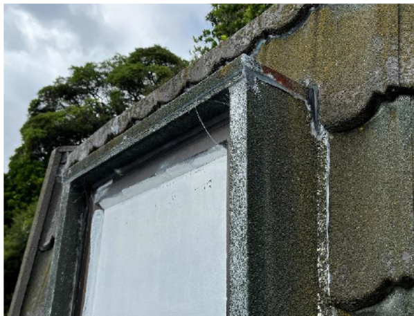
2.4 There are numerous failed sealant repairs to prevent moisture ingress into the building.
