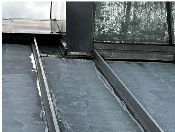
1.76 Open flashing and glazing joint between the roof and lantern
