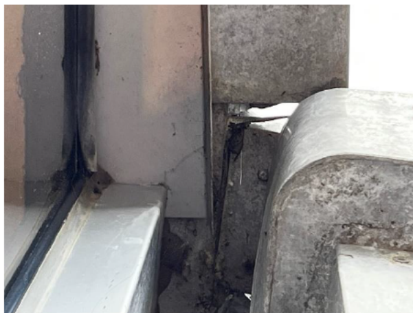
1.158 Gap between the gutter and rain head
