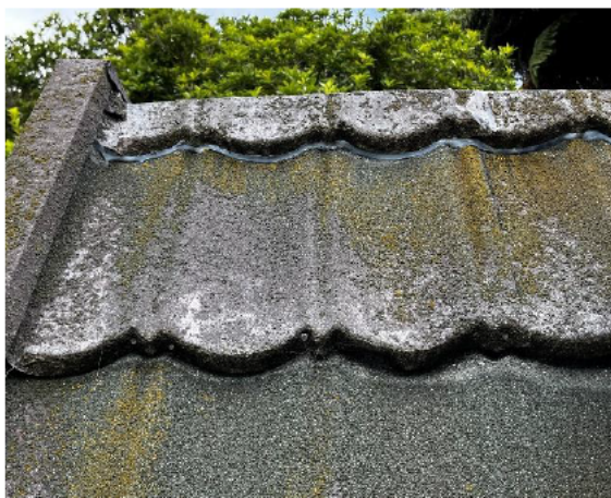
2.5 Sealant repairs at the hip junction
