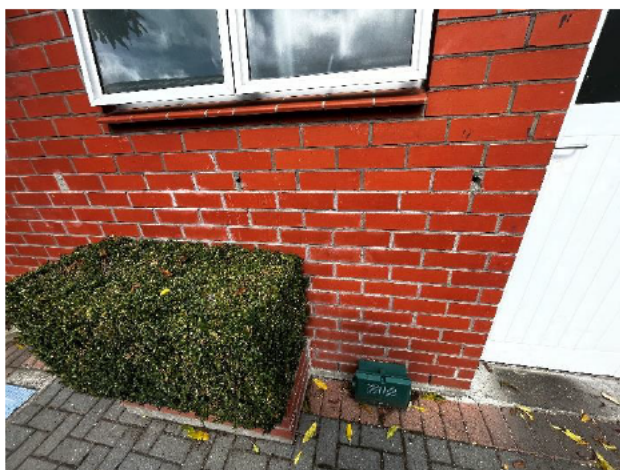
2.41 Unsealed obsolete penetration holes through the wall
