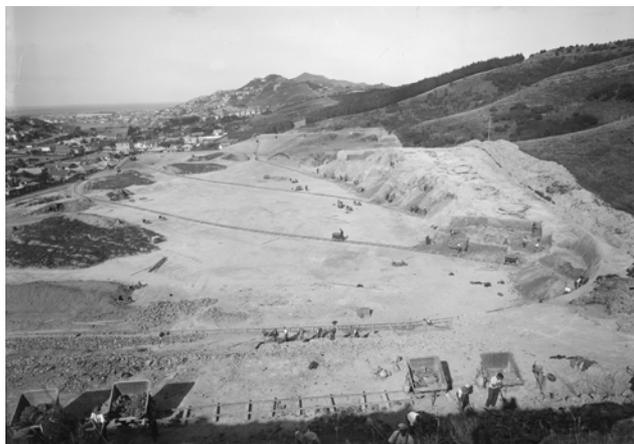
*Hataitai Park under construction in 1932. Relief labour dug out banks and moved spoil in metal bins on rails. Spoil from the Mount Victoria tunnel was also used to form the park.
